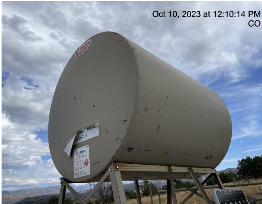
Photo # 2291 Methanol tank lacks required information
