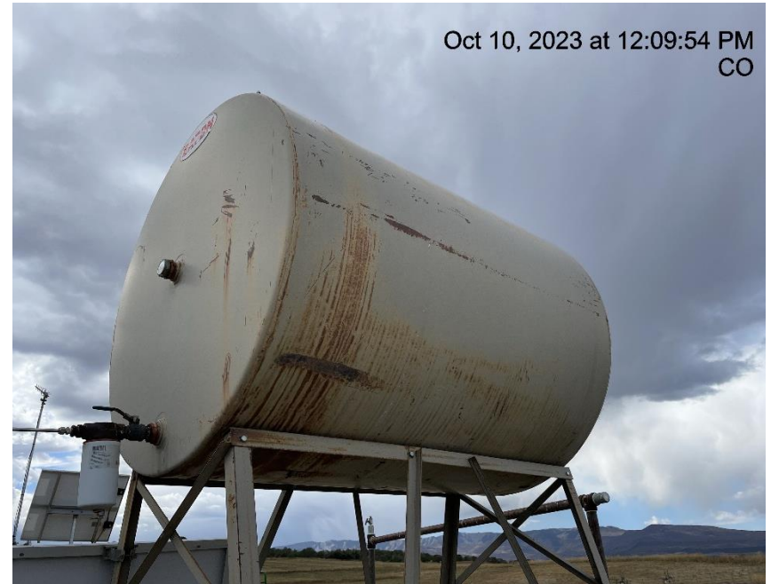
Photo # 2292 Methanol tank lacks required information
