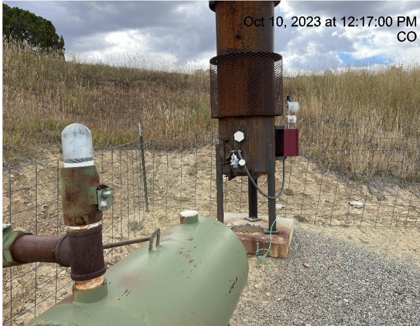
Photo # 2295 Unused equipment/ECD is disconnected
