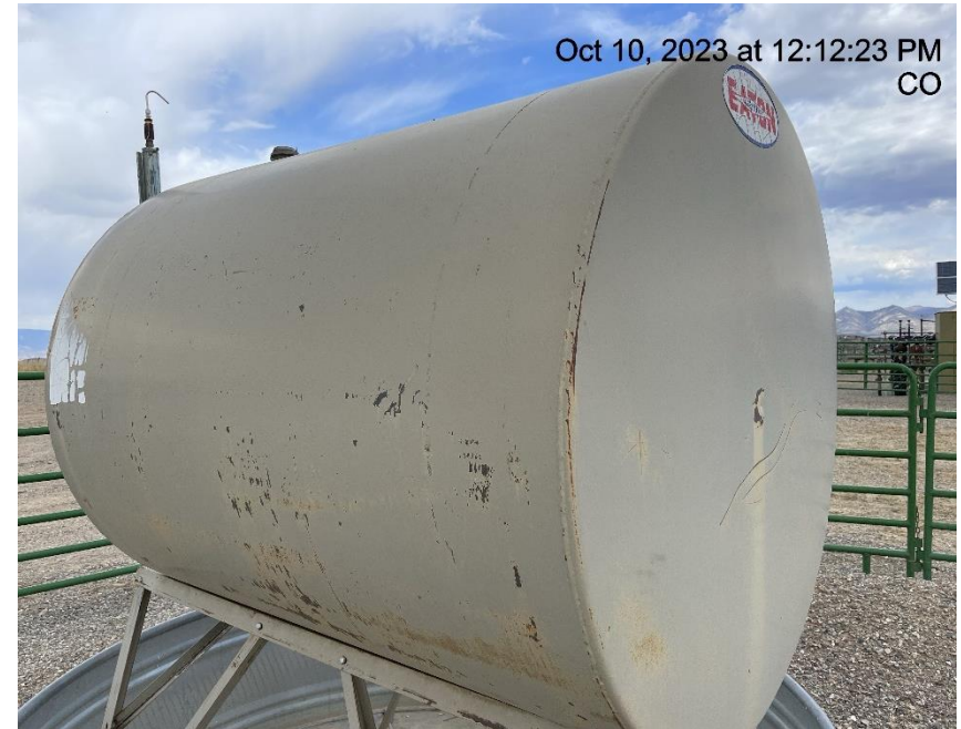
Photo # 2294 Methanol tank lacks required information
