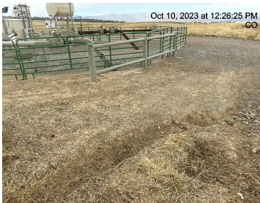
Photo # 2315 Erosion & transport of sediment off location
