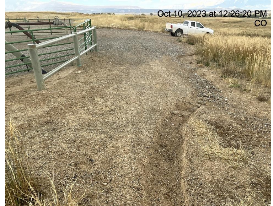
Photo # 2314 Erosion & transport of sediment off location
