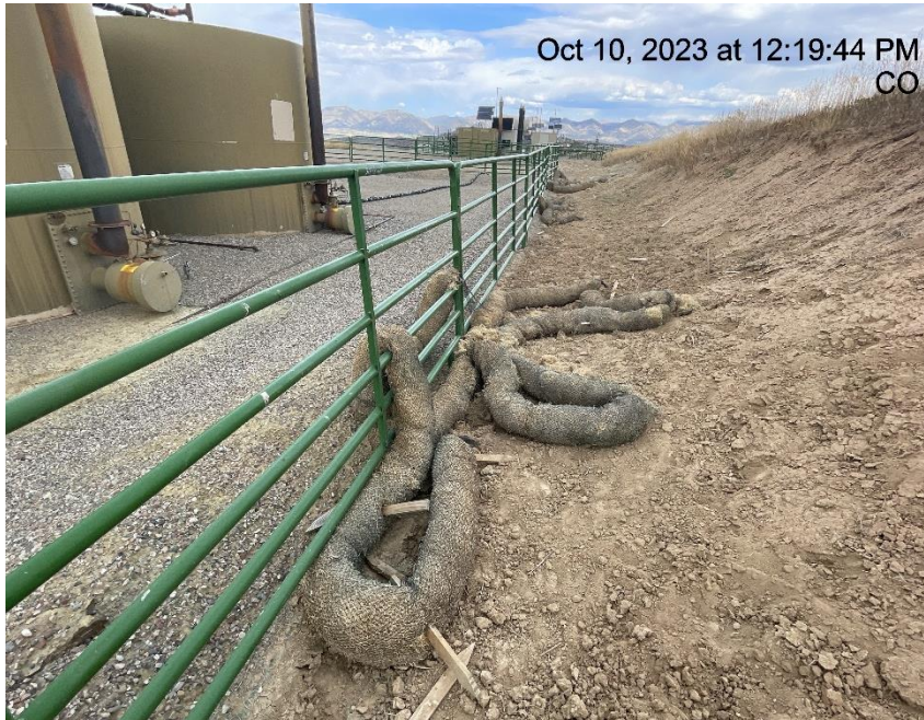
Photo # 2309 Erosion/lack of stabilization on slope
