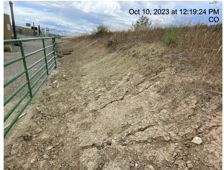
Photo # 2306 Erosion/lack of stabilization on slope
