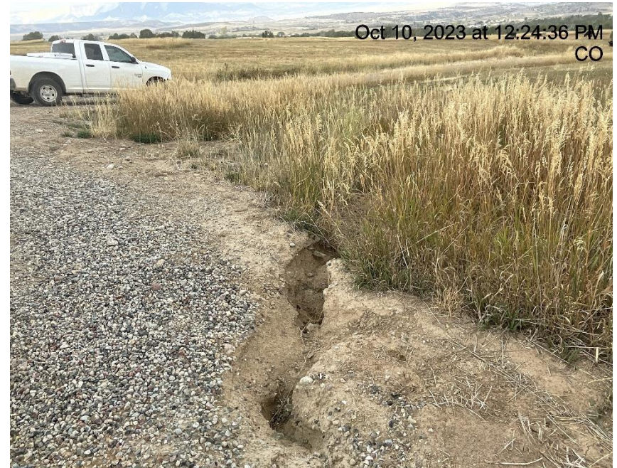
Photo # 2310 Erosion & transport of sediment off location
