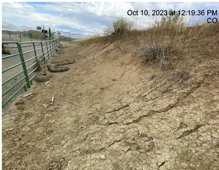
Photo # 2307 Erosion/lack of stabilization on slope
