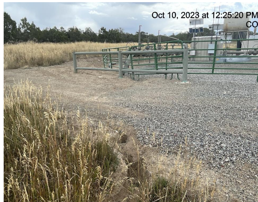
Photo # 2312 Erosion & transport of sediment off location
