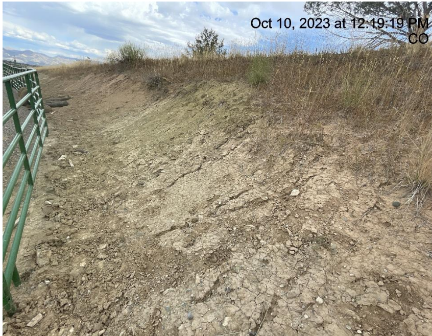
Photo # 2305 Erosion/lack of stabilization on slope
