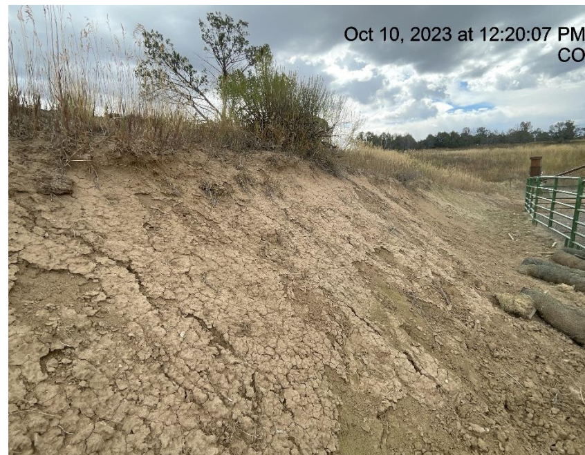
Photo # 2308 Erosion/lack of stabilization on slope
