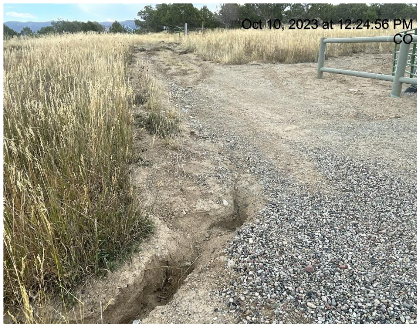
Photo # 2311 Erosion & transport of sediment off location
