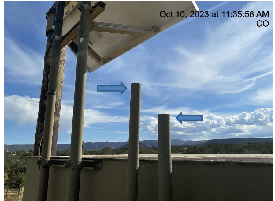
Photo # 2215 PRV & rupture disk vent lines lack caps
