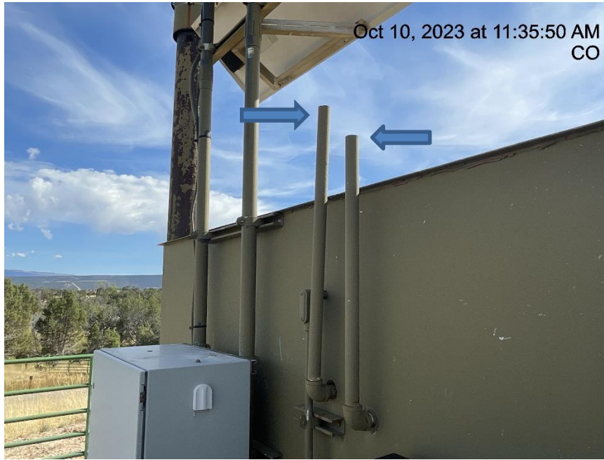
Photo # 2214 PRV & rupture disk vent lines lack caps
