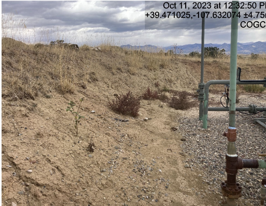
Cut slope erosion
