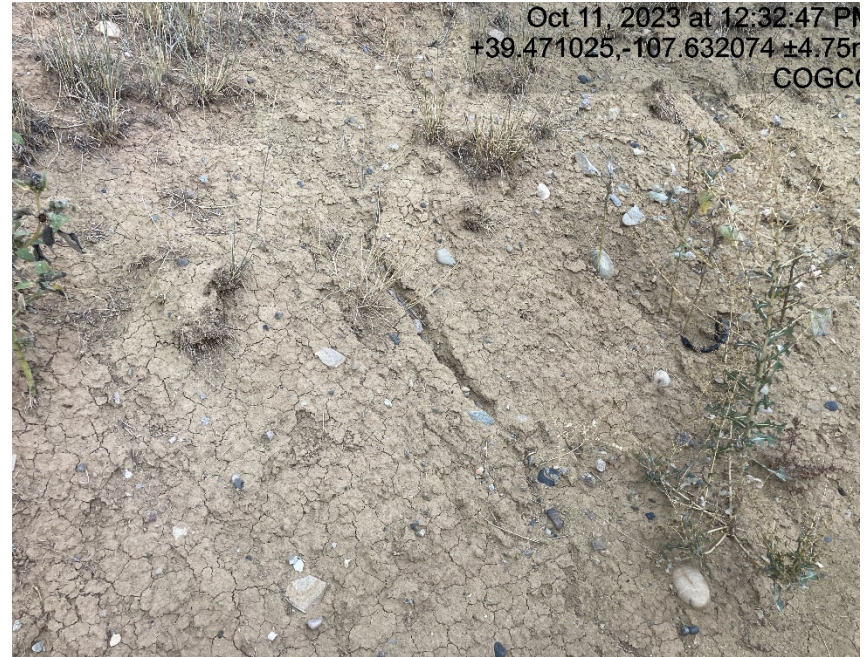
Cut slope erosion
