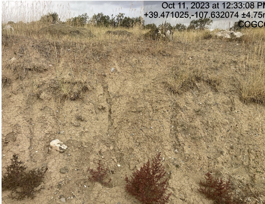
Cut slope erosion
