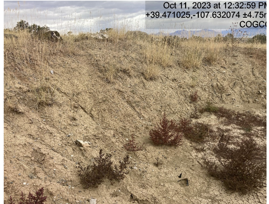
Cut slope erosion
