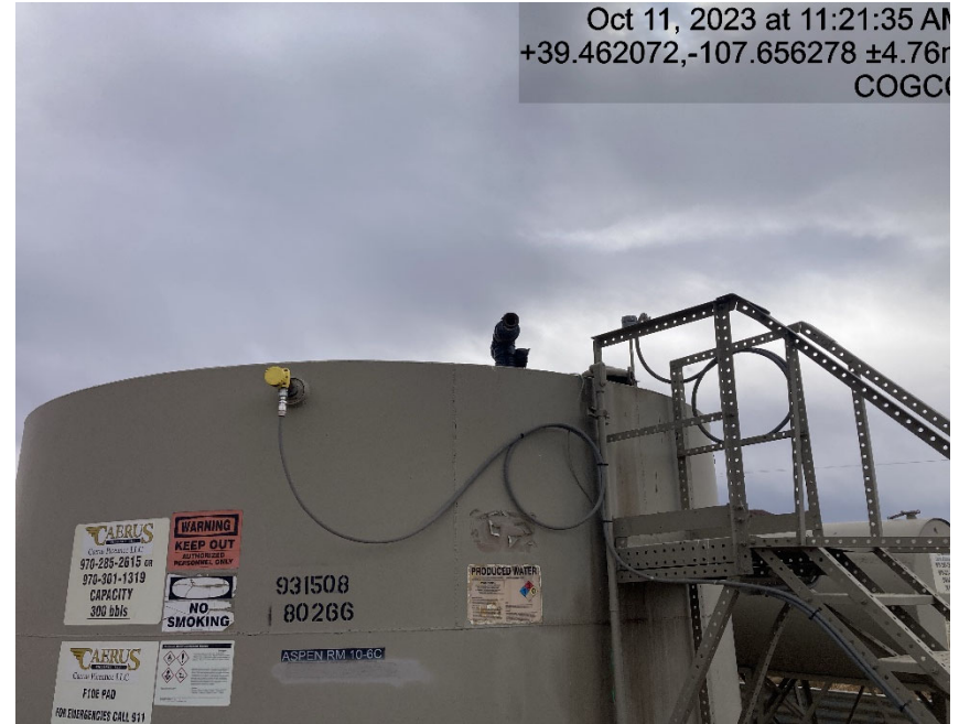
Line on tank is open for wildlife to enter
