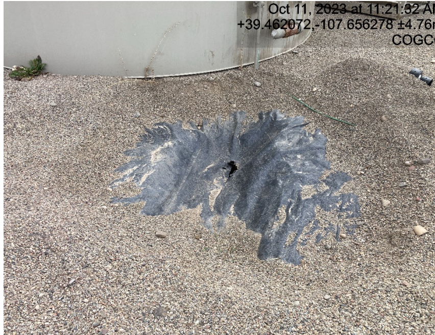
Hole in containment and some debris
