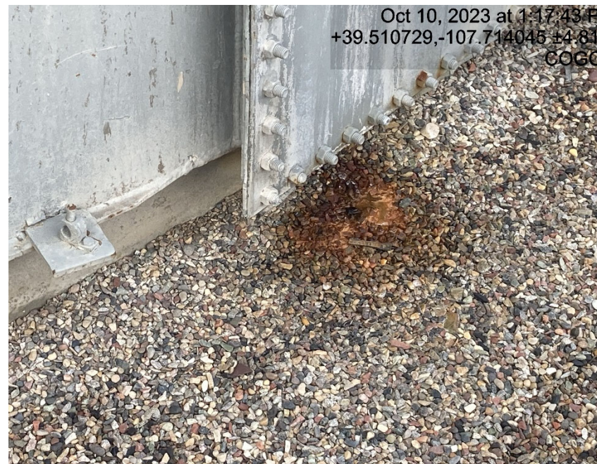
Leaking tank
