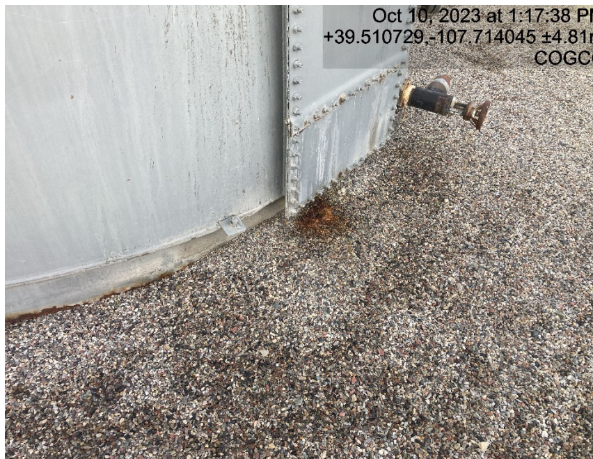
Leaking tank
