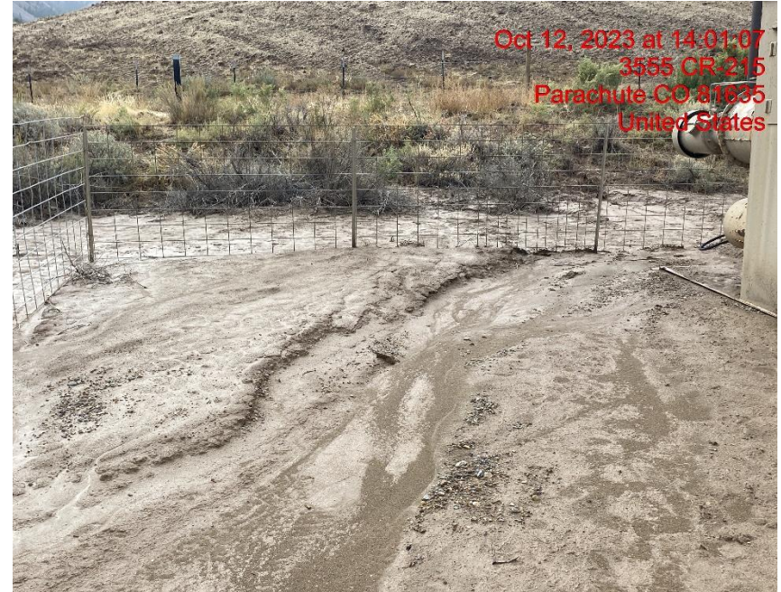
Insufficient Erosion Control/Sediment Run-on to Location – Photo #06906
