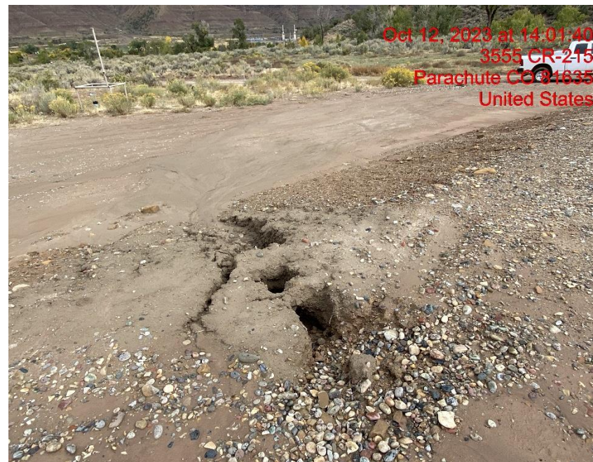
Insufficient Erosion Control – Photo #06908
