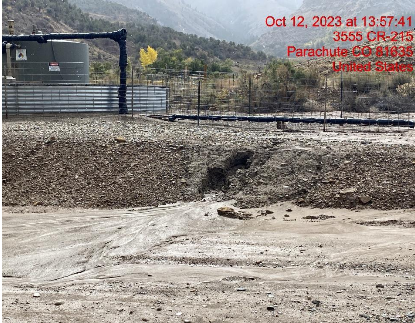
Insufficient Erosion Control – Photo #06901
