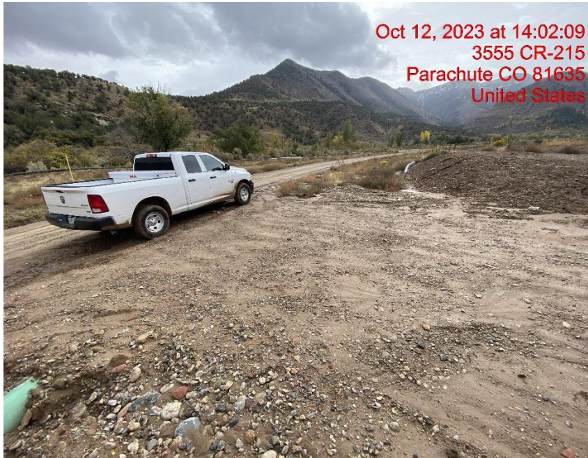
Insufficient Vehicle Tracking BMPs at Location Entrance/Exit – Photo #06909
