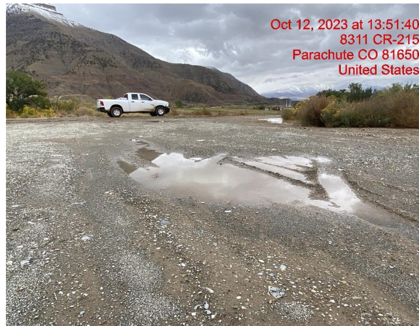
Location Lacks Stabilization – Photo #06897
