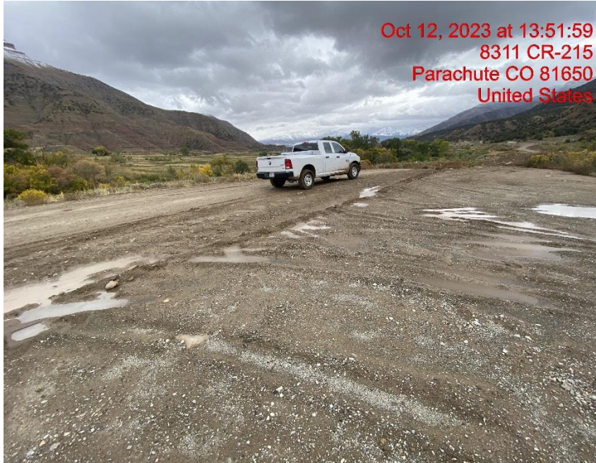
Insufficient Vehicle Tracking BMPs at Location Entrance/Exit – Photo #06898
