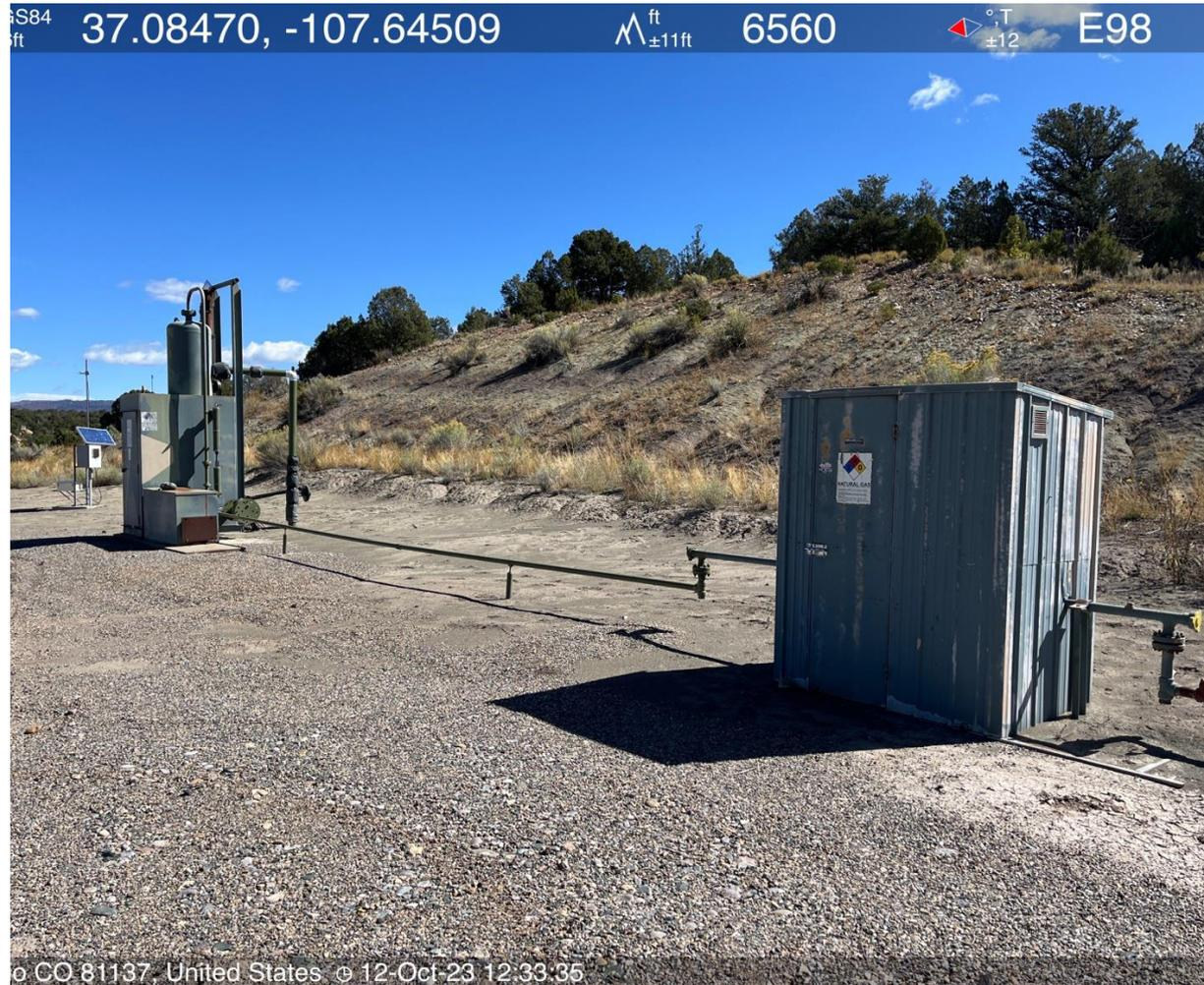
Photo #4 View of the separator, meterhouse, and telemetry.
