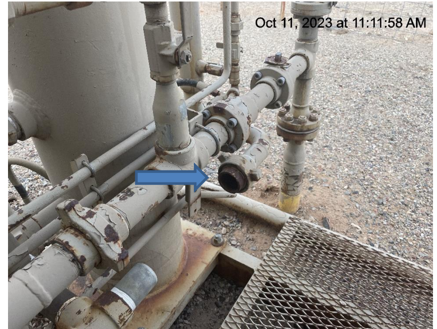
Photo # 2374 Open ended pipe/wildlife hazard
