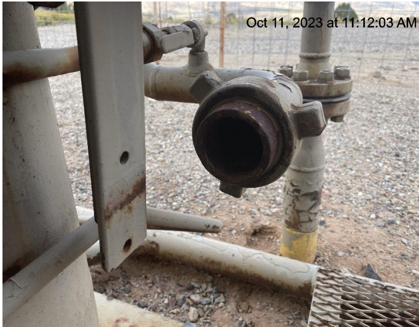
Photo # 2375 Open ended pipe/wildlife hazard
