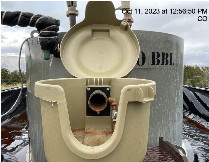
Photo # 2508 Open ended load line
