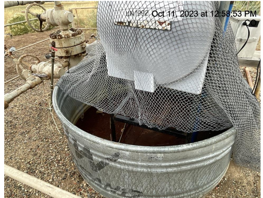
Photo # 2507 Netting/Wildlife protection needs maintenance
