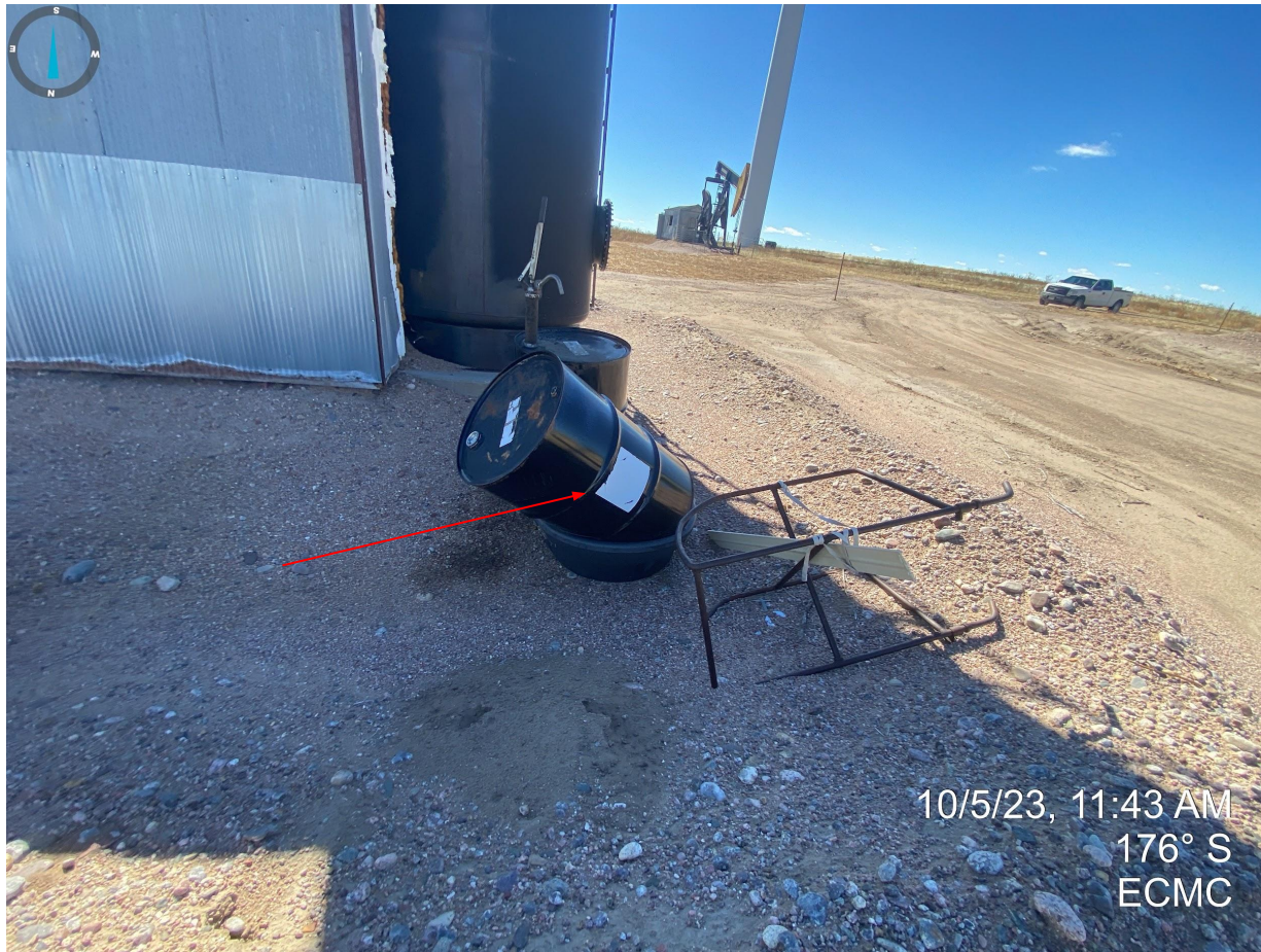
Photo 3. Drum not within adequate secondary containment.
