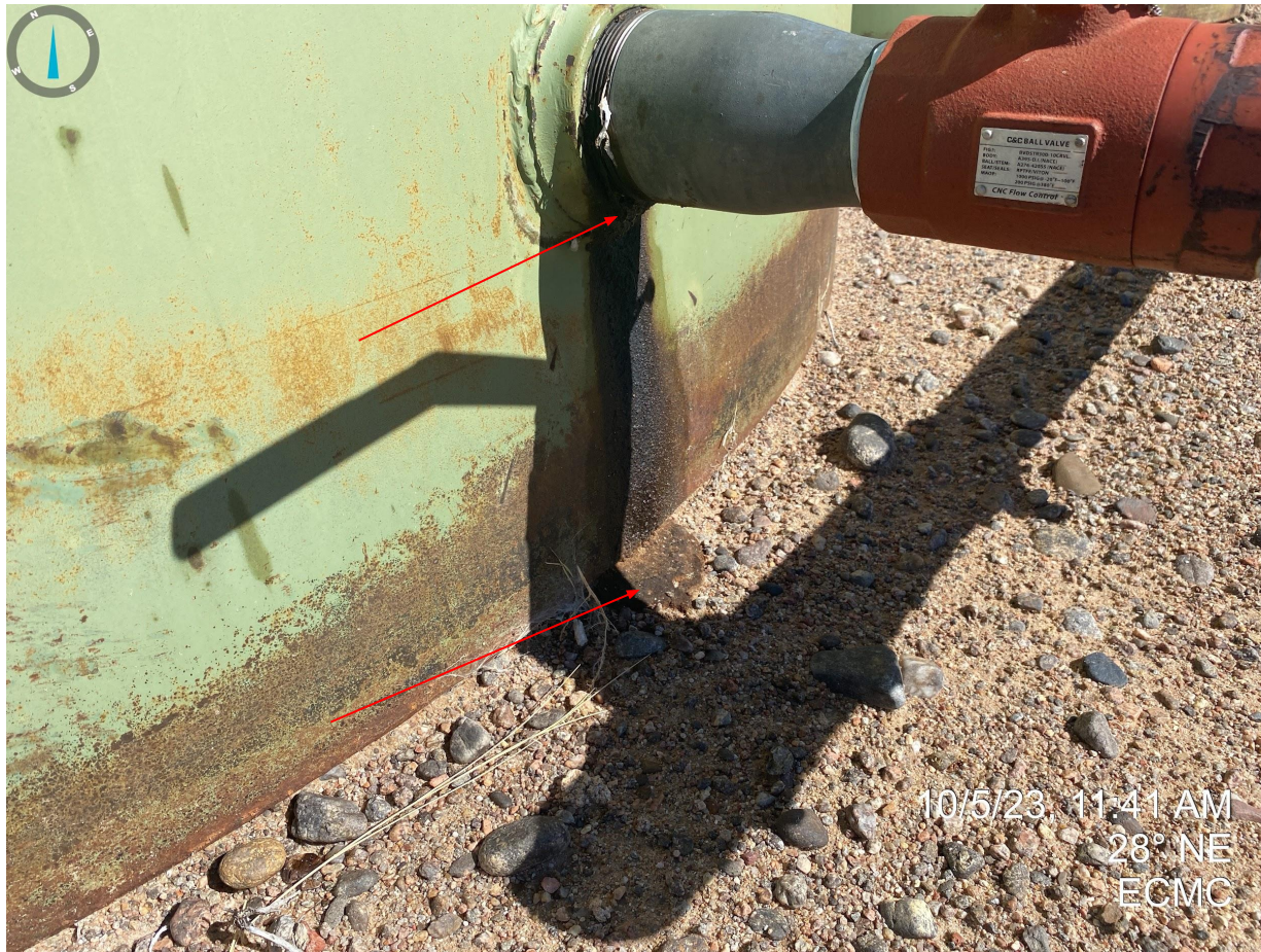
Photo 2. Stained soil and leaking equipment/fitting at tank battery.
