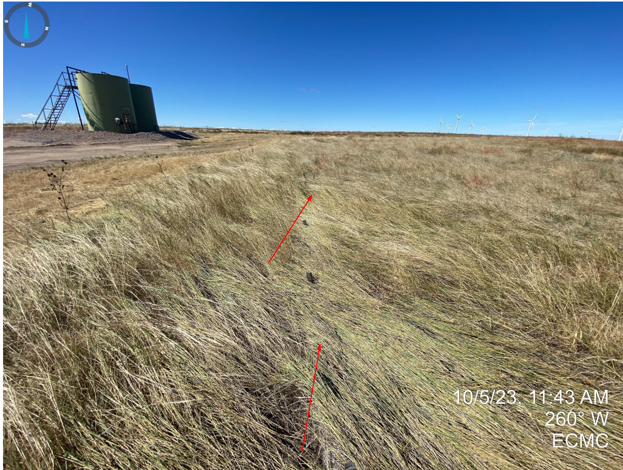
Photo 5. Degraded straw wattles are now considered debris and need to be removed.
