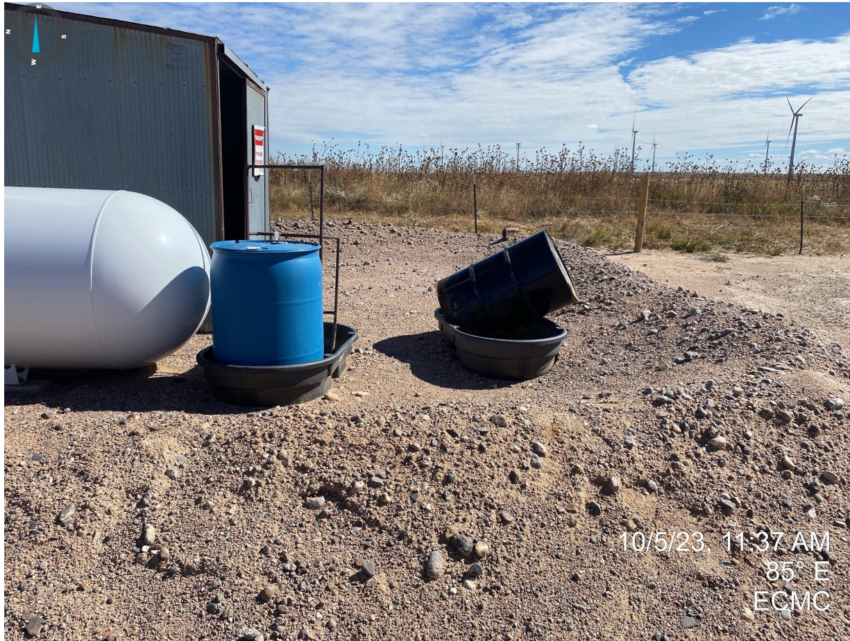
Photo 26. Unmarked/labeled drums within inadequate secondary containment, and no wildlife exclusion devices (e.g. netting) observed around secondary containment.
