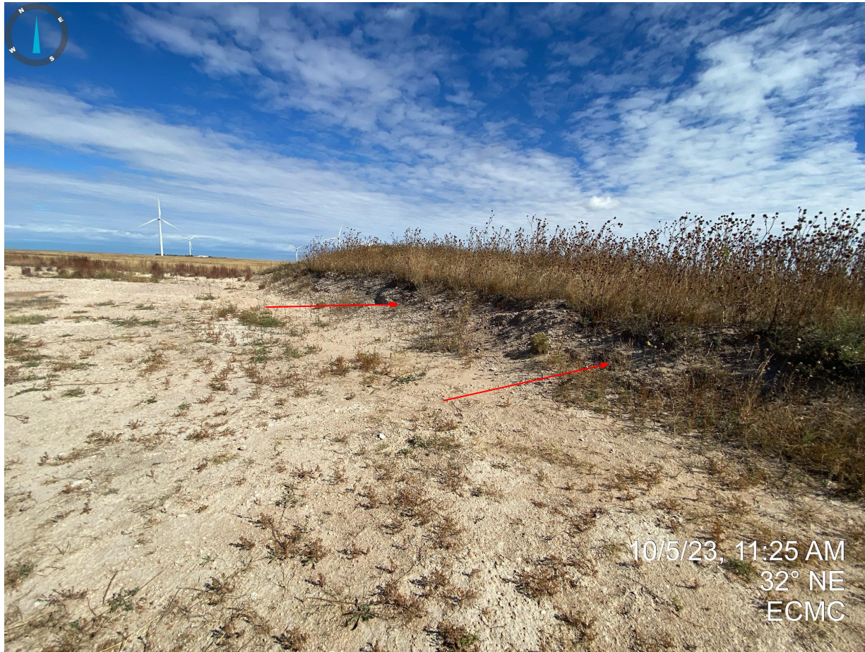
Photo 10. The western edge of the topsoil stockpile is not properly stabilized with evidence of wind/water erosion observed.
