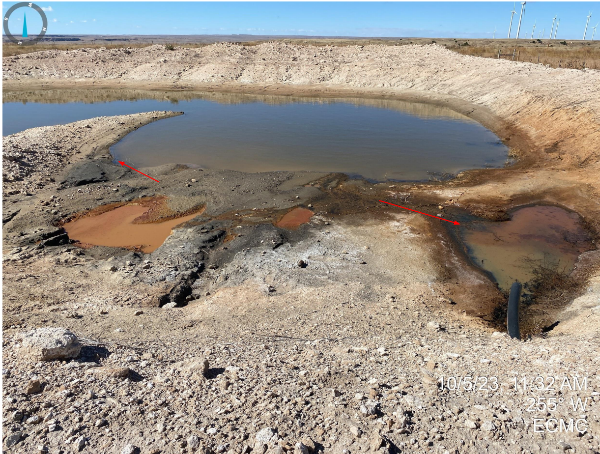
Photos 23-25. Hydrocarbon impacts observed within the pit.
