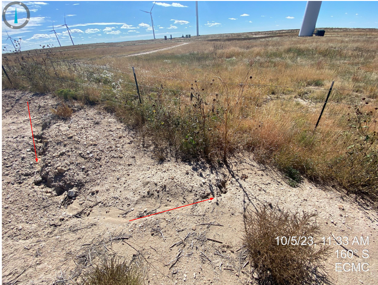
Photo 22. Erosion degradation occurring from the pit berms/walls.
