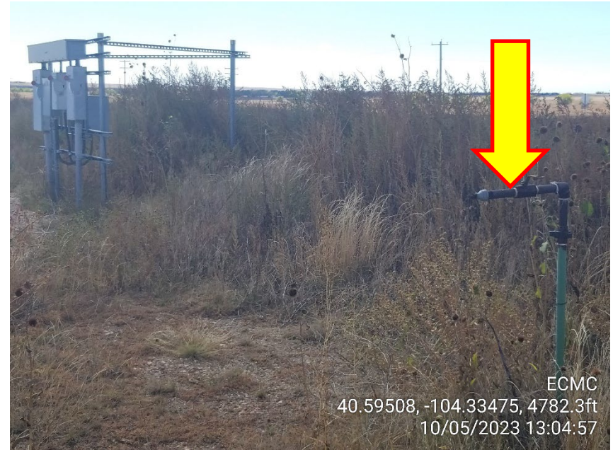
Photo 14 – Unmarked Riser
