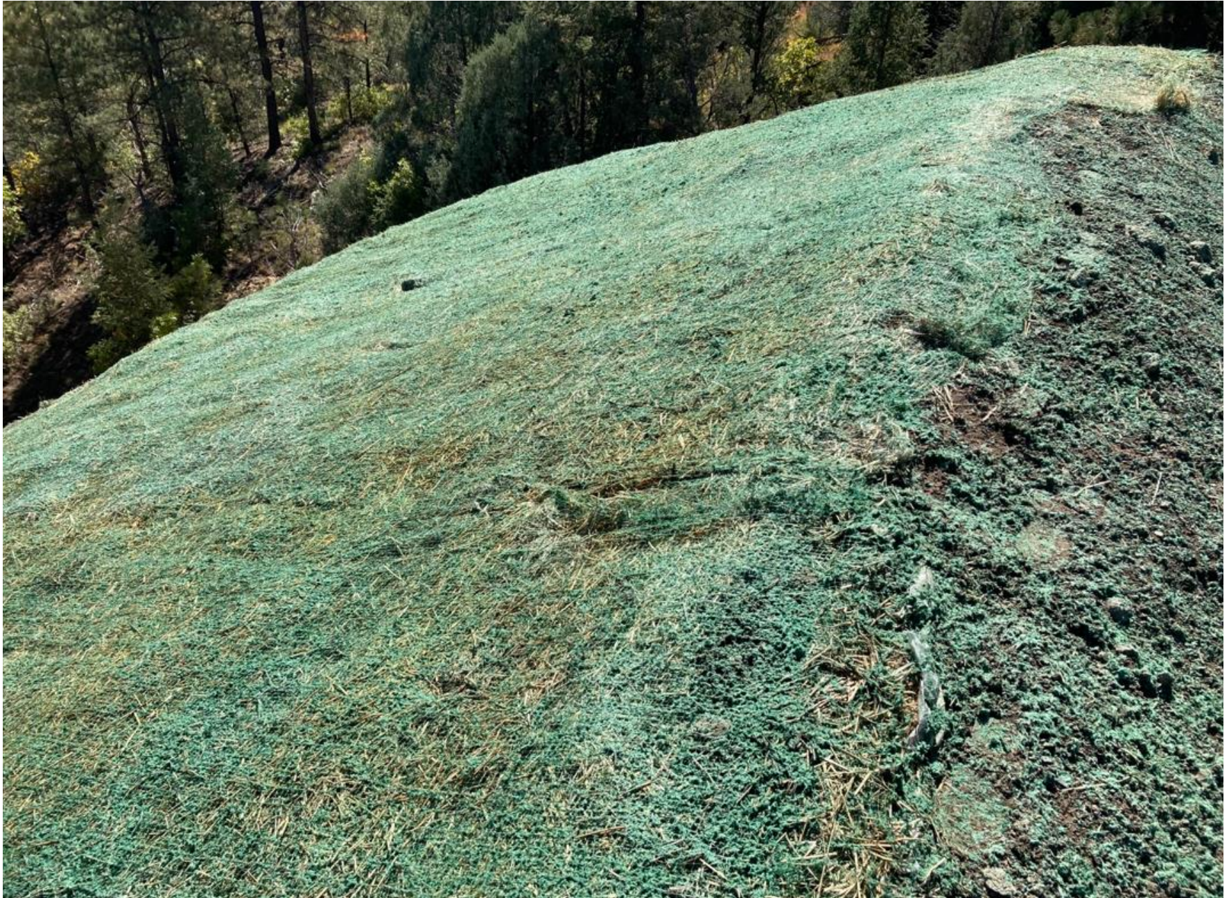
PHOTO 3: STRAW BLANKETS WERE INSTALLED OVER THE ENTIRE FILL SLOPE. ALL DISTIRBED AREAS WERE TRACKED, SEEDED, AND HYDROMULCHED TO FURTHER PROMOTE STABILIZATION THROUGH VEGETATIVE GROWTH.
