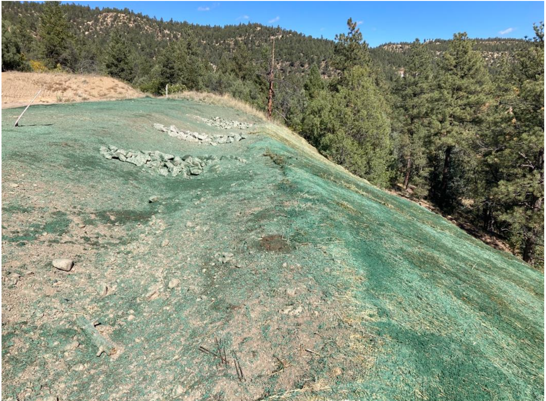
PHOTO 2: A DIVERSION DITCH WAS CREATED ALONG THE TOP OF THE FILL SLOPE TO DIRECT STORM WATER OFF LOCATION AND PREVENT RILLING ON THE SLOPE. ROCK CHECK DAMS WERE INSTALLED TO CONTROL RUN ON VELOCITY.
