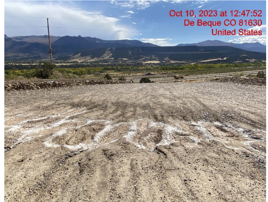
Insufficient Vehicle Tracking BMPs at Location Entrance/Exit – Photo #06860
