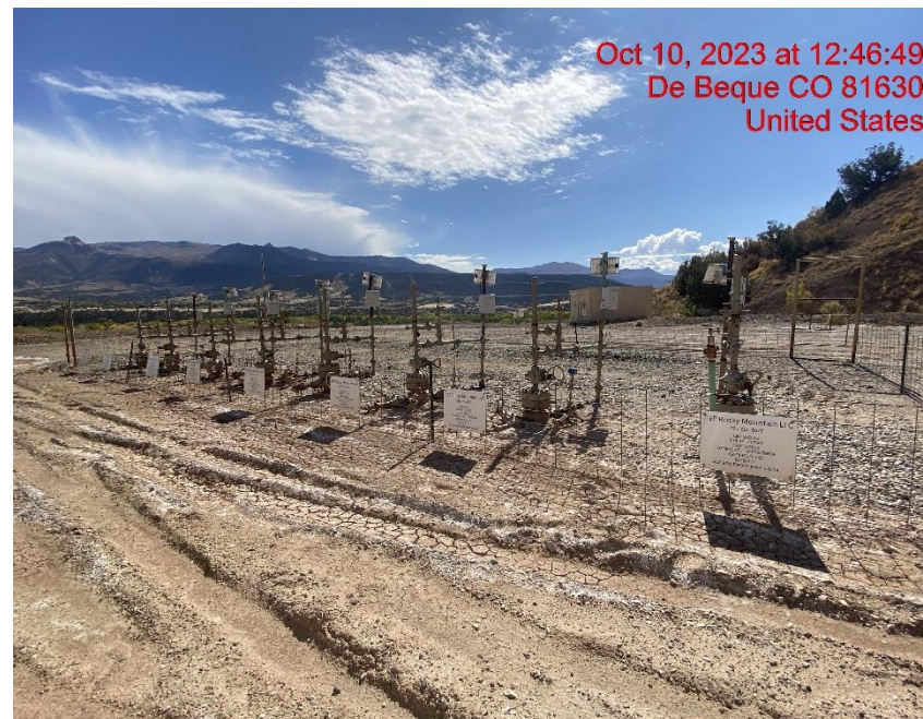
Wellheads/Lack of Stabilization – Photo #06857
