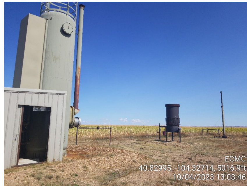
Photo 4 – Heater Treater, ECD and Flare
