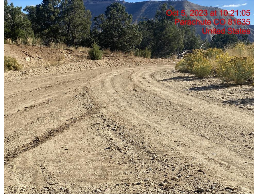
Insufficient Vehicle Tracking BMPs at Location Entrance/Exit – Photo #06835
