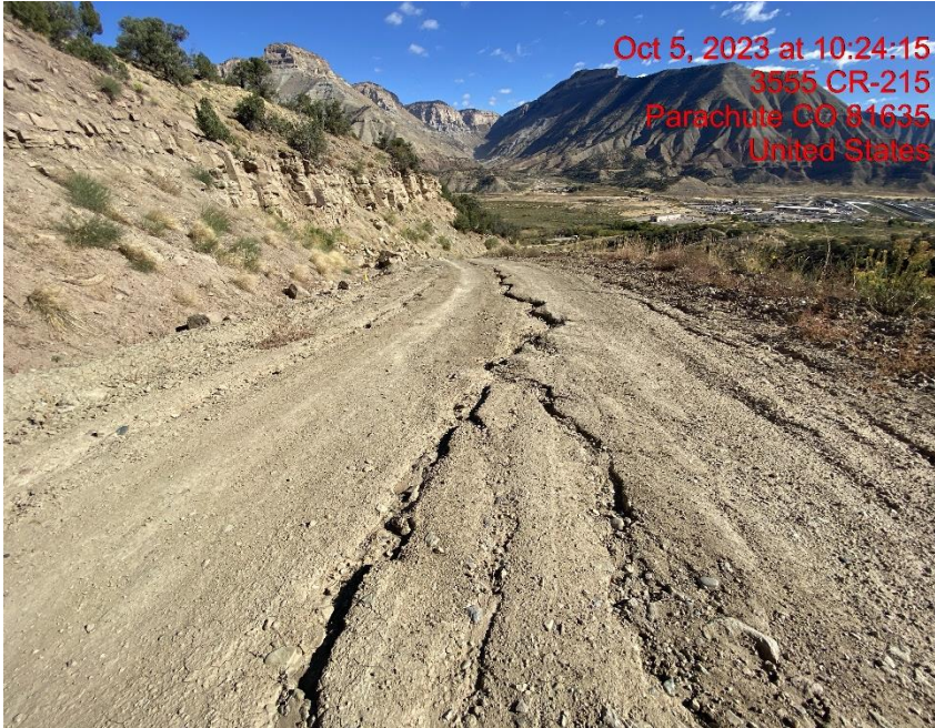
Insufficient Erosion Controls/Rill Erosion on Lease Road – Photo #06836
