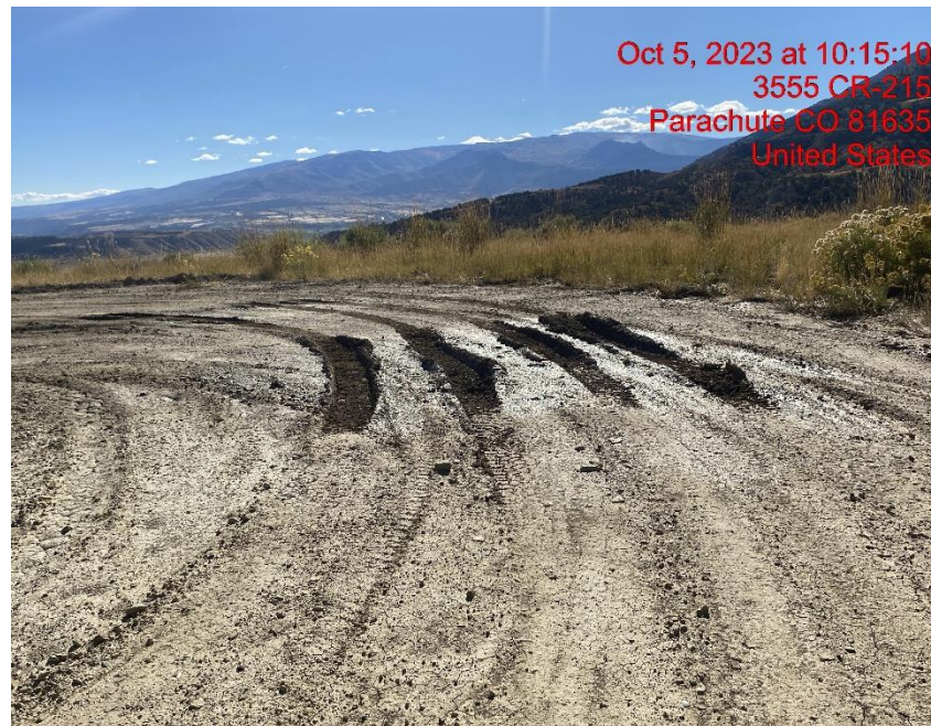
Location Lacks Stabilization – Photo #06827
