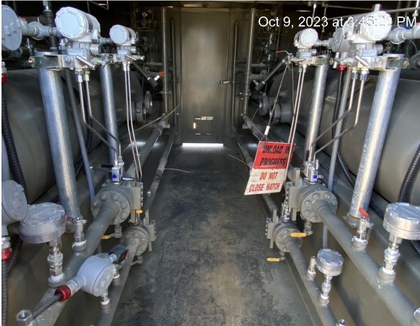
No visible display of gas meter calibration at each meter
