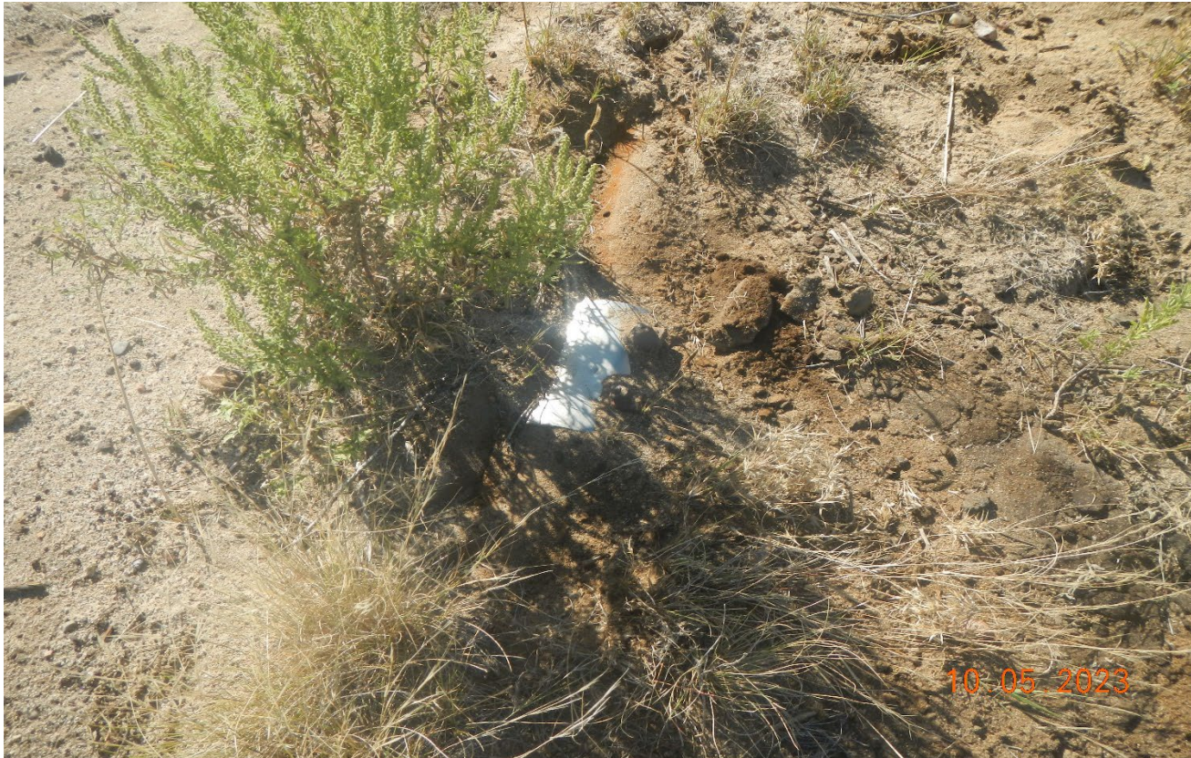
Photo 3. There is an exposed flowline at the surface that needs to be removed. . Lat/Long:38.42686,-102.46158.
