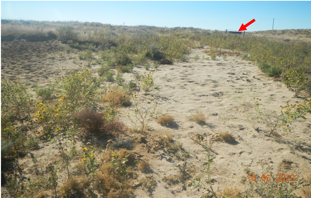
Photo 8. Facing southwest at the abandoned wellsite location. The sandy soils have not revegetated and need to be seeded and reclaimed. The red arrow points to the abandoned flowline cellar that needs to be removed.
