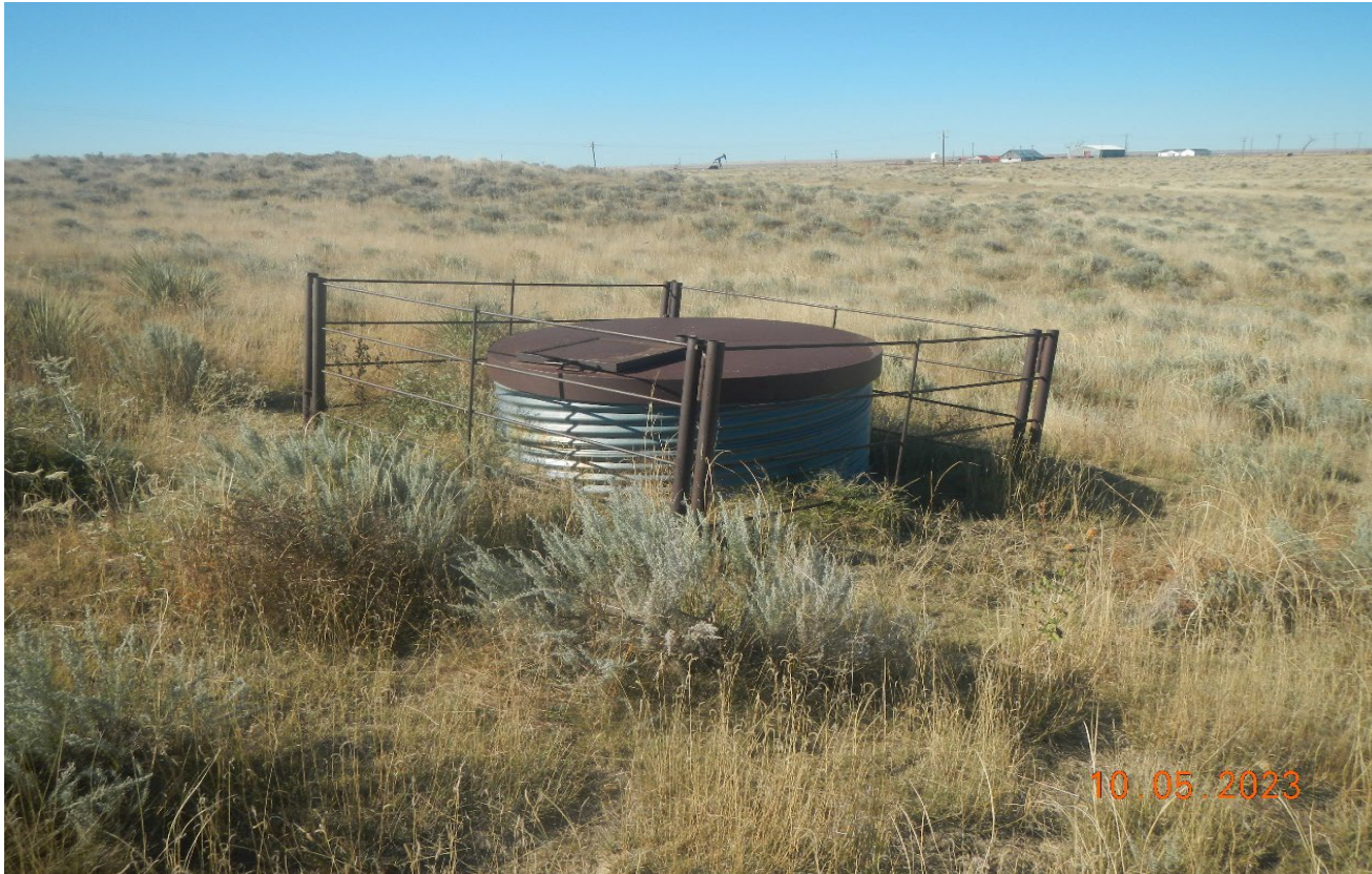
Photo 5. Facing southwest near the abandoned wellsite is abandoned flowline cellar that needs to be removed. Lat/Long:38.42706, -102.46211.
