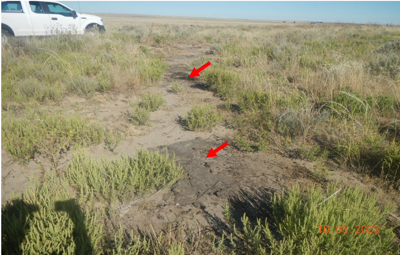
Photo 1. Facing northwest along the abandoned flowline near the location. There is oily sludge shown at red arrow that needs to be cleaned up. Lat/Long:38.42686,-102.46158.
