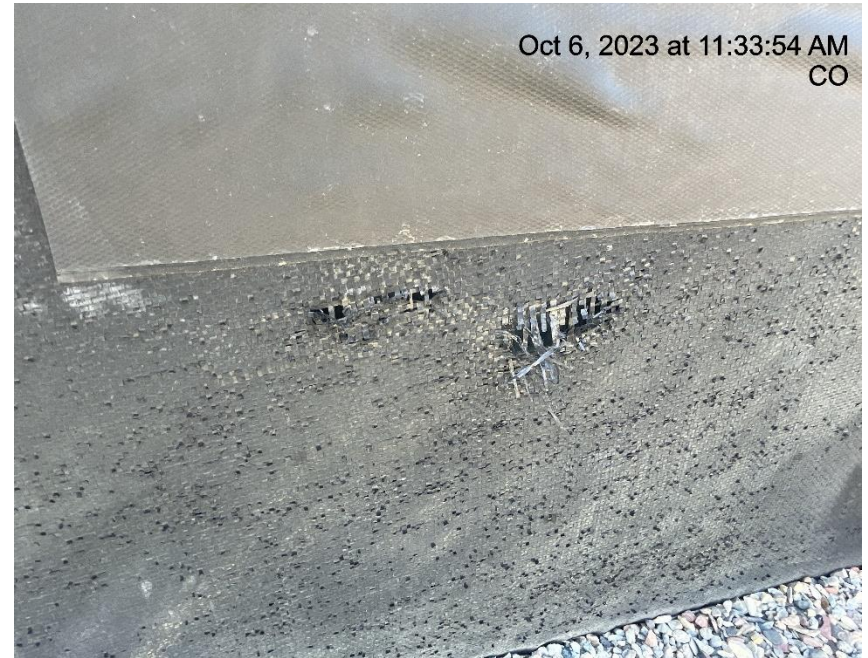
Photo # 1927 Hole in secondary containment liner/liner needs maintenance
