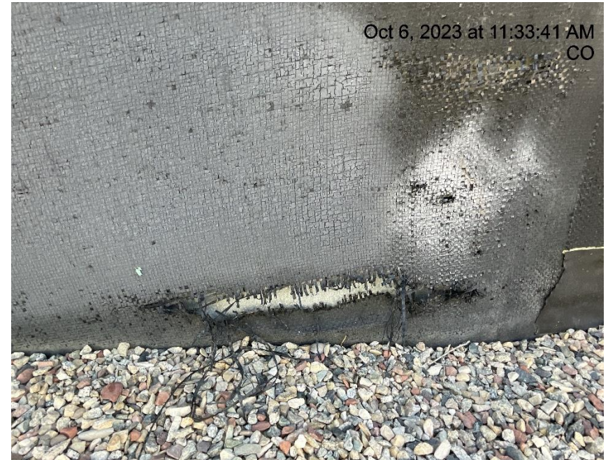
Photo # 1925 Hole in secondary containment liner/liner needs maintenance
