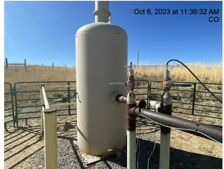
Photo # 1931 Unused equipment/ECD disconnected
