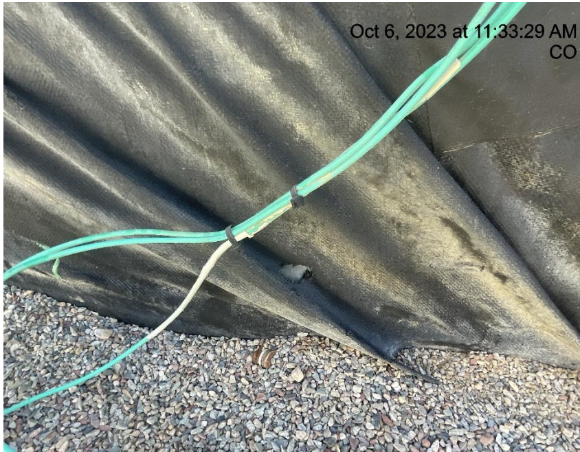
Photo # 1926 Hole in secondary containment liner/liner needs maintenance
