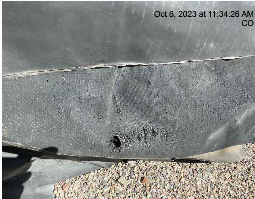
Photo # 1928 Hole in secondary containment liner/liner needs maintenance
