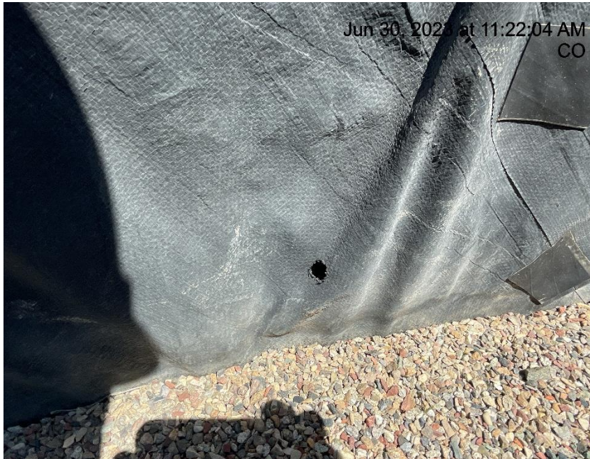
Photo # 2272 From inspection 708900904 conducted on 06/30/2023 Hole in secondary containment liner/liner needs maintenance
