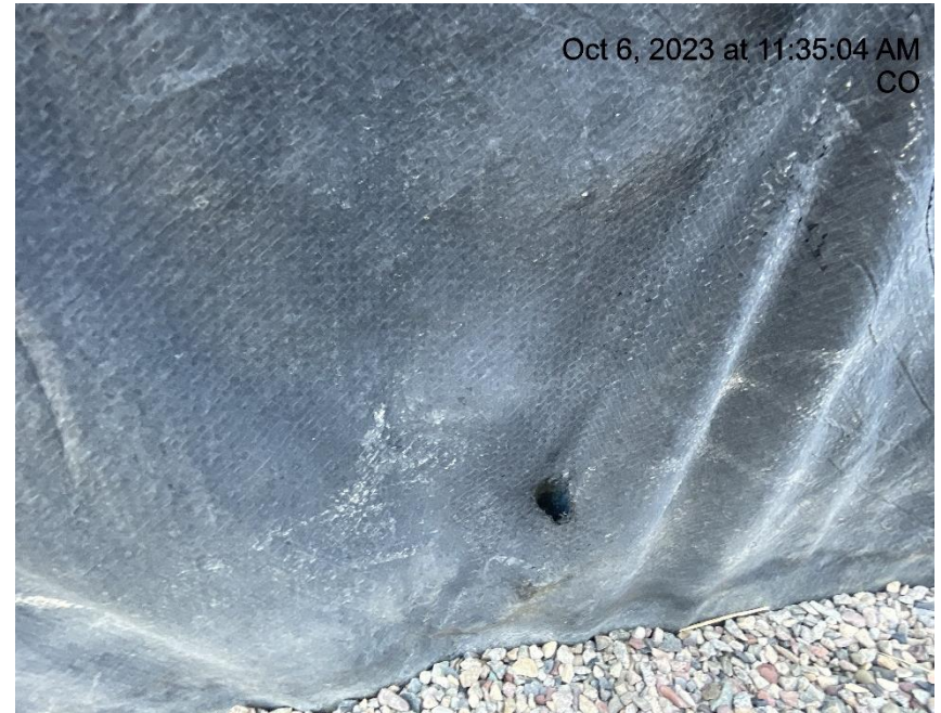
Photo # 1922 Hole in secondary containment liner/liner needs maintenance
