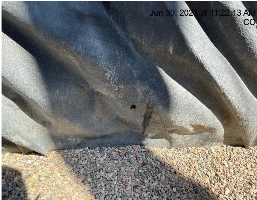
Photo # 2274 From inspection 708900904 conducted on 06/30/2023 Hole in secondary containment liner/liner needs maintenance
