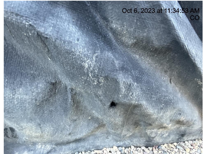
Photo # 1923 Hole in secondary containment liner/liner needs maintenance
