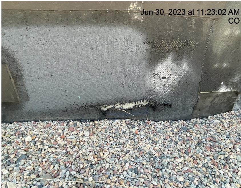
Photo # 2282 From inspection 708900904 conducted on 06/30/2023 Hole in secondary containment liner/liner needs maintenance
