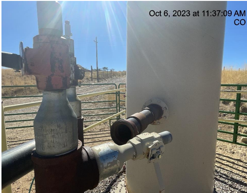
Photo # 1932 Unused equipment/ECD disconnected
