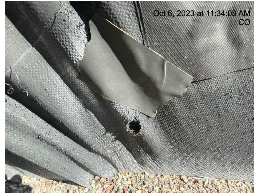
Photo # 1924 Hole in secondary containment liner/liner needs maintenance
