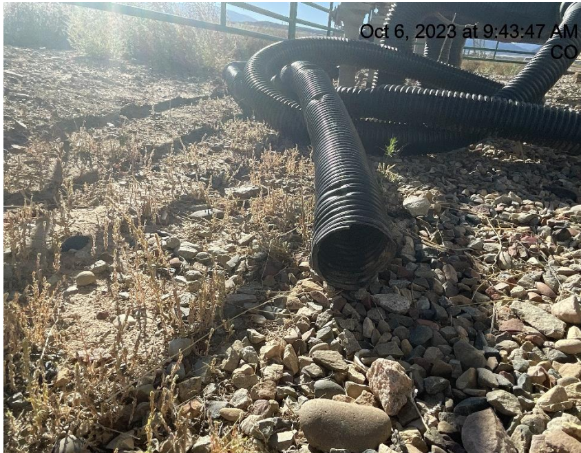
Photo # 1800 Flowline heating insulation open ended
