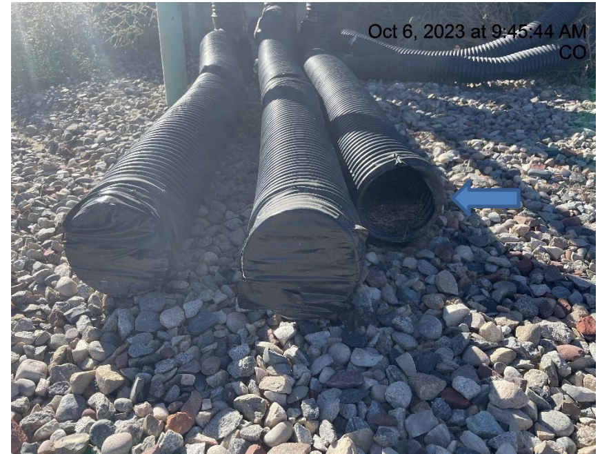
Photo # 1801 Flowline heating insulation open ended
