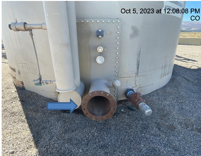
Photo # 1730 Burner tube on production tank open ended/wildlife hazard
