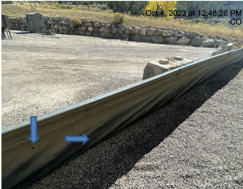
Photo # 1582 Holes in liner/liner needs maintenance
