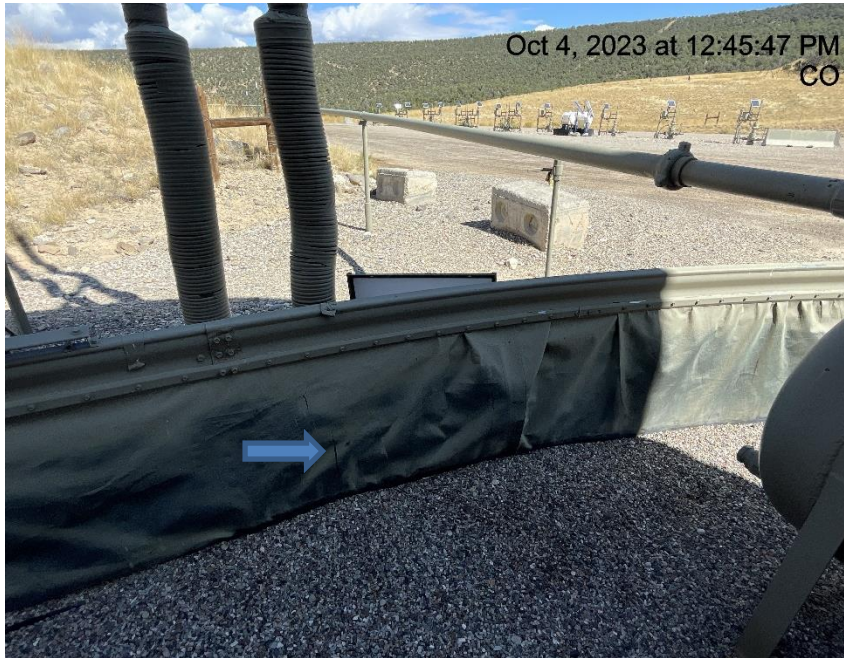
Photo # 1578 Hole in liner/liner needs maintenance
