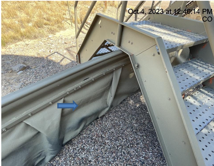
Photo # 1580 Hole in liner/liner needs maintenance
