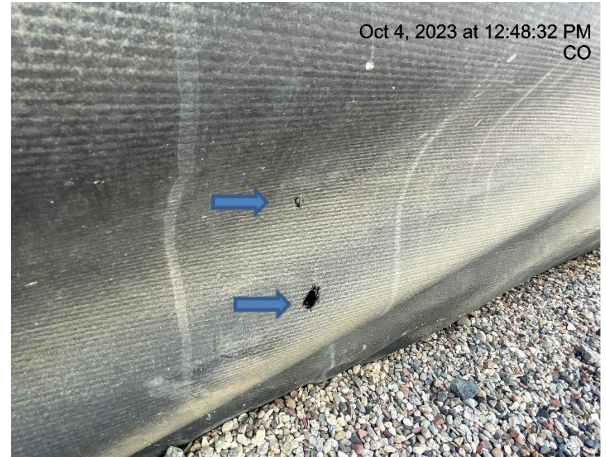
Photo # 1583 Holes in liner/liner needs maintenance
