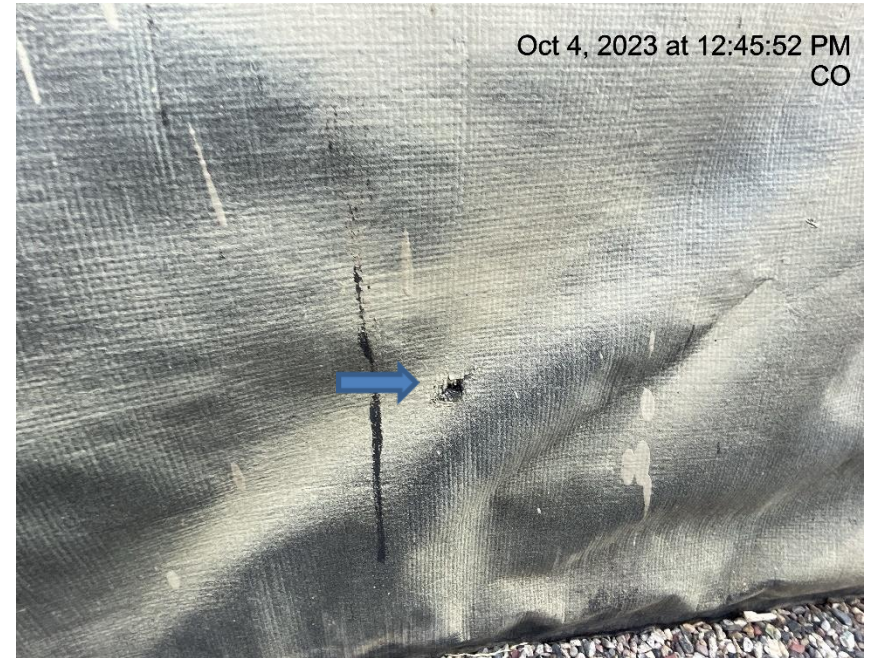
Photo # 1579 Hole in liner/liner needs maintenance
