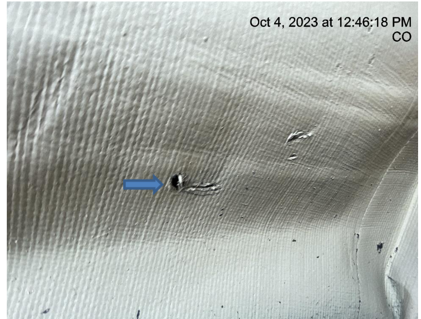
Photo # 1581 Hole in liner/liner needs maintenance
