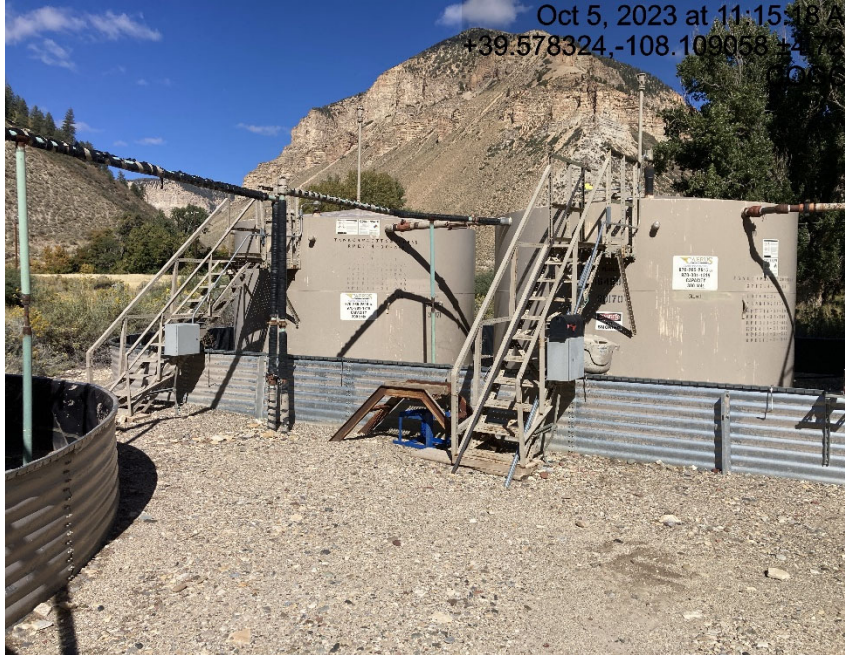
Tank battery lacking signage
