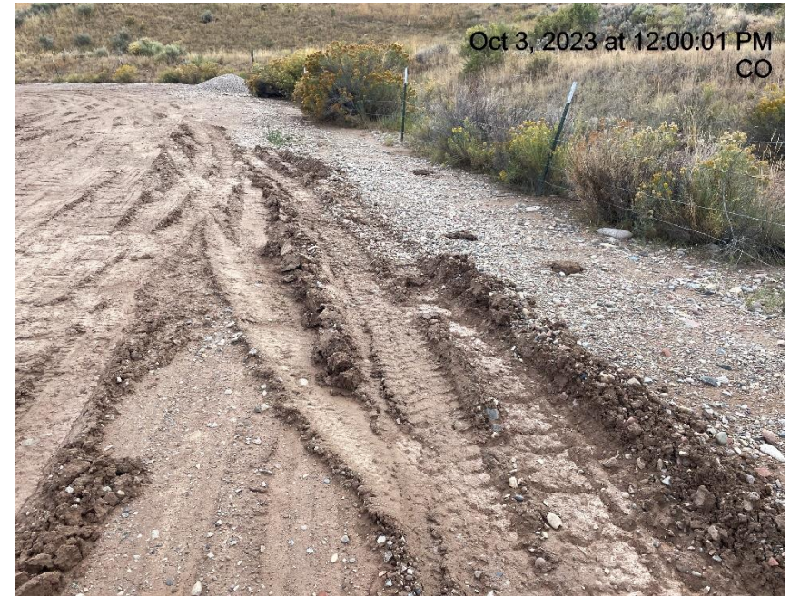
Photo # 1365 Lack of stabilization/compaction/insufficient BMP's
