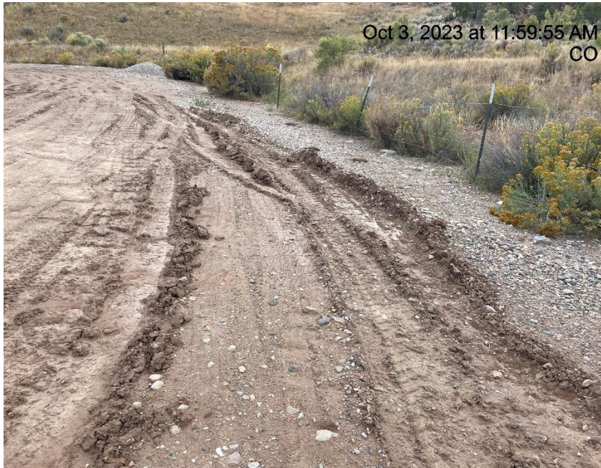
Photo # 1364 Lack of stabilization/compaction/insufficient BMP's
