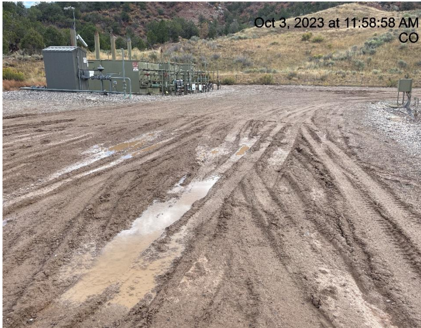
Photo # 1362 Lack of stabilization/compaction/insufficient BMP's
