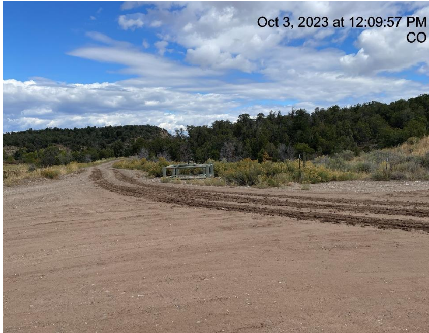
Photo # 1372 Vehicle tracking onto lease road/insufficient tracking BMP's
