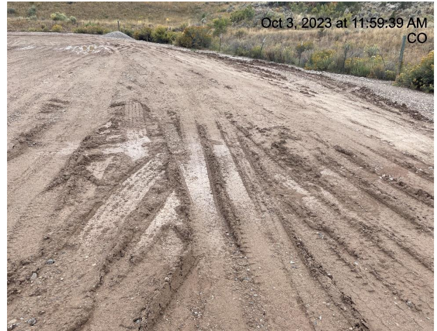
Photo # 1363 Lack of stabilization/compaction/insufficient BMP's
