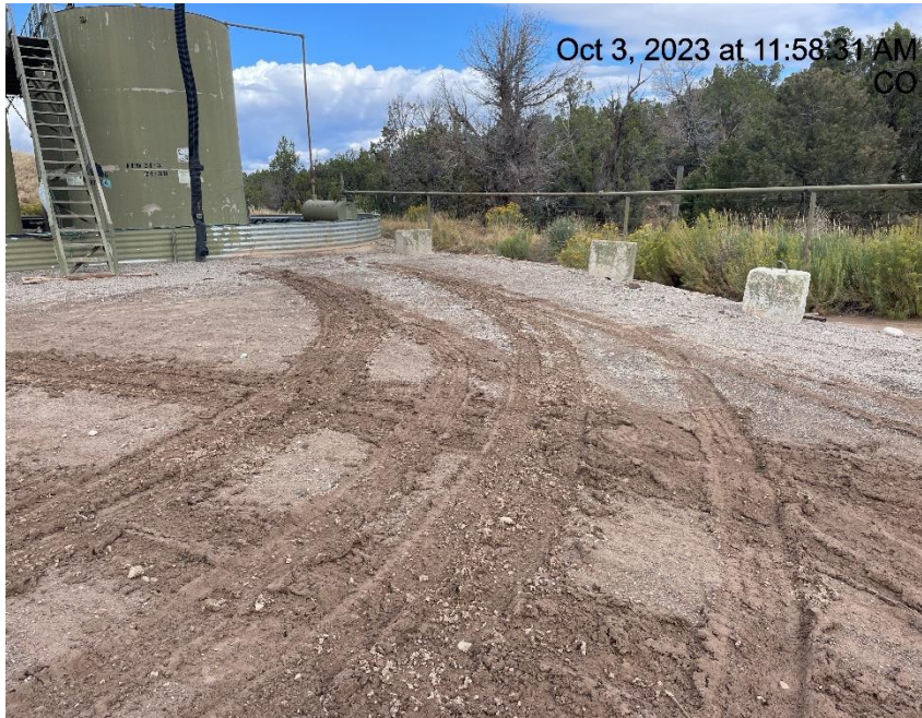
Photo # 1360 Lack of stabilization/compaction/insufficient BMP's
