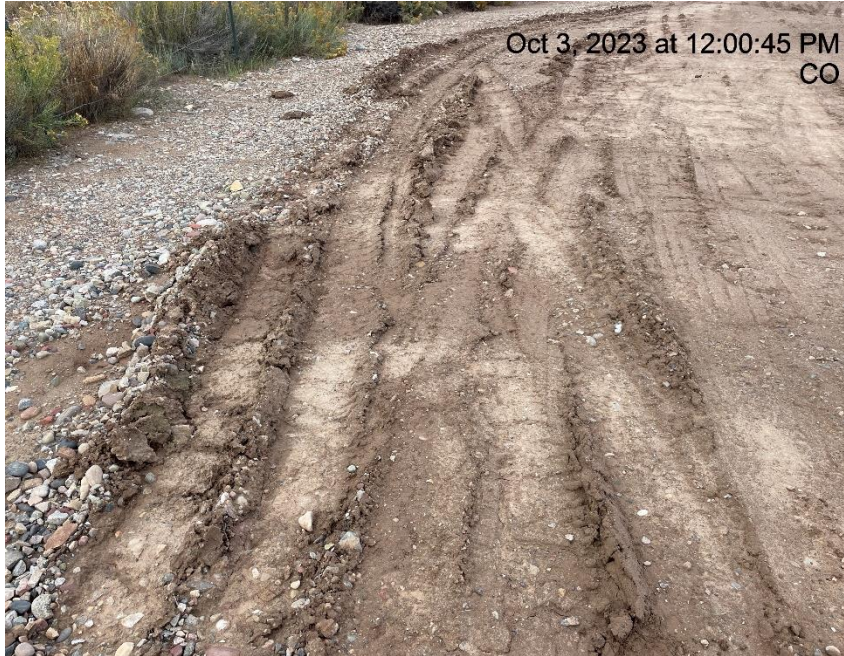
Photo # 1366 Lack of stabilization/compaction/insufficient BMP's
