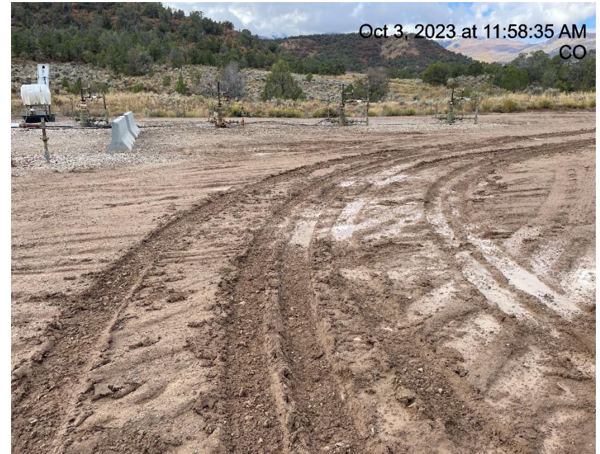
Photo # 1361 Lack of stabilization/compaction/insufficient BMP's
