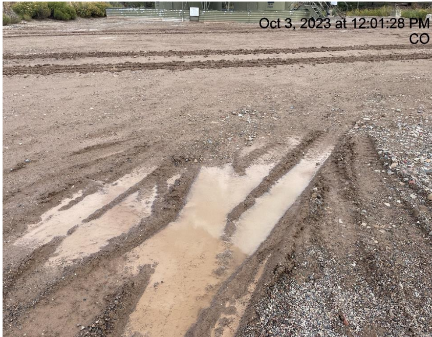
Photo # 1368 Lack of stabilization/compaction/insufficient BMP's
