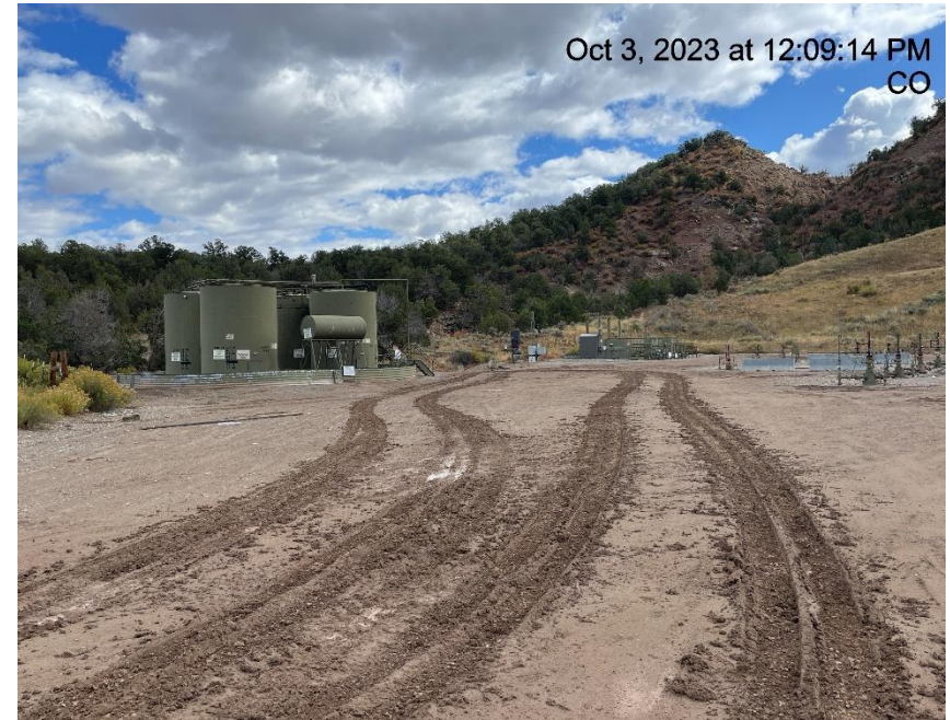
Photo # 1369 Lack of stabilization/compaction/insufficient BMP's
