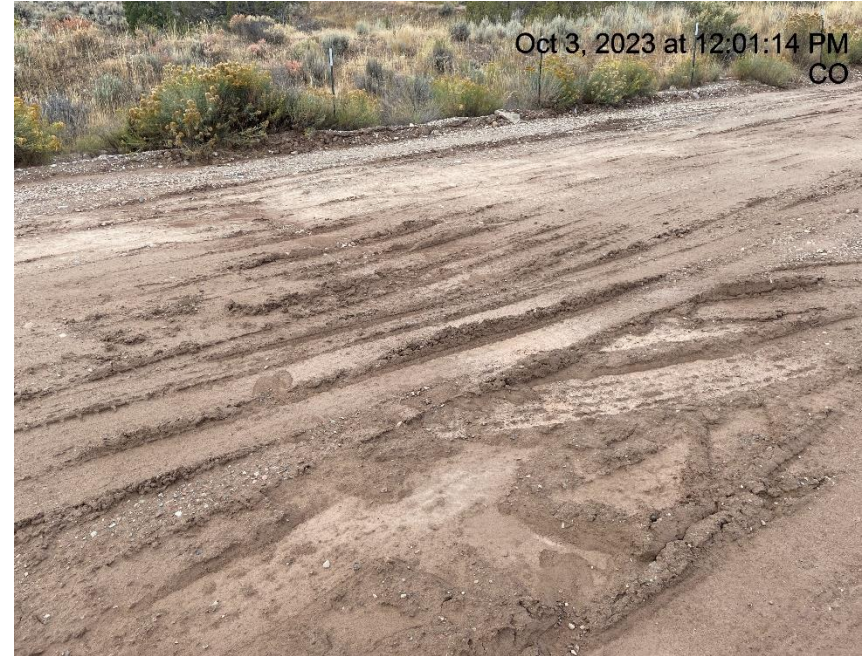
Photo # 1367 Lack of stabilization/compaction/insufficient BMP's
