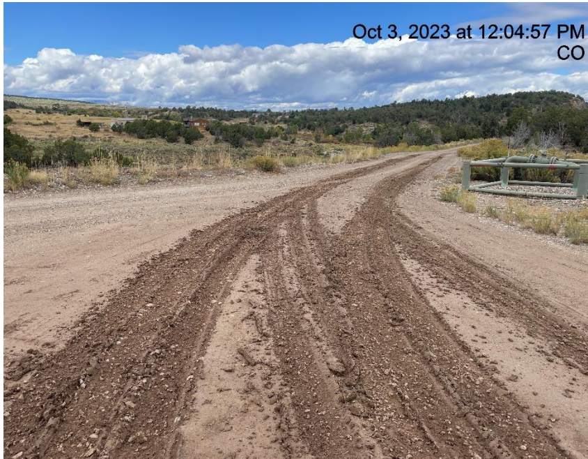
Photo # 1376 Vehicle tracking onto lease road/insufficient tracking BMP's
