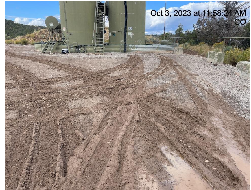
Photo # 1359 Lack of stabilization/compaction/insufficient BMP's
