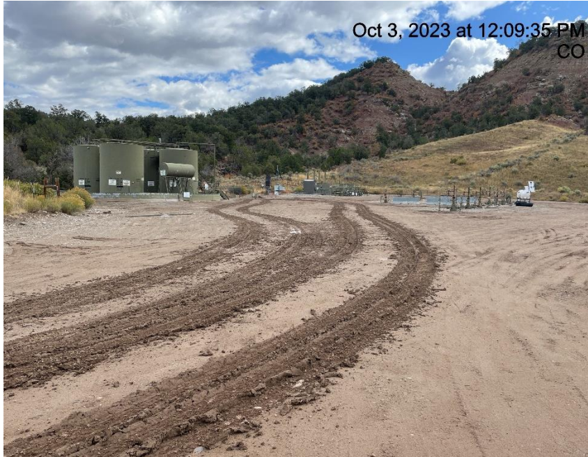
Photo # 1370 Lack of stabilization/compaction/insufficient BMP's
