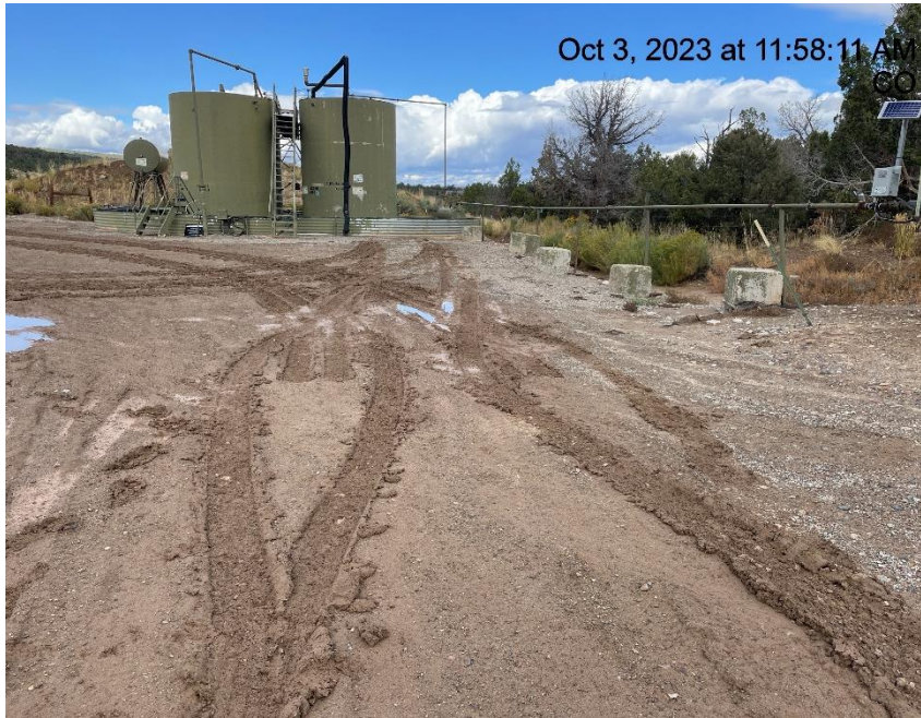
Photo # 1358 Lack of stabilization/compaction/insufficient BMP's
