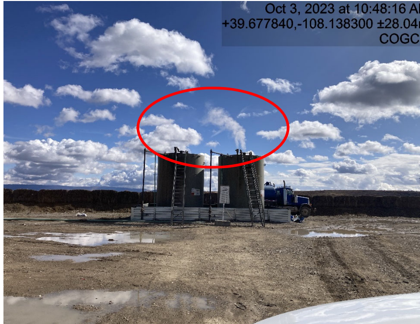
Tank battery and venting from thief hatch and PRV
