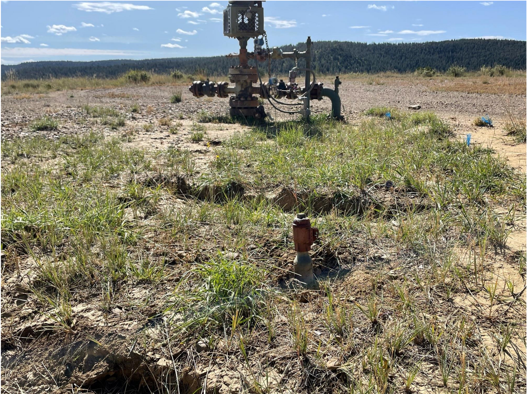
PHOTO 2: THE RISER HAS BEEN PLUGGED AND MARKED, PER RULE 606.
