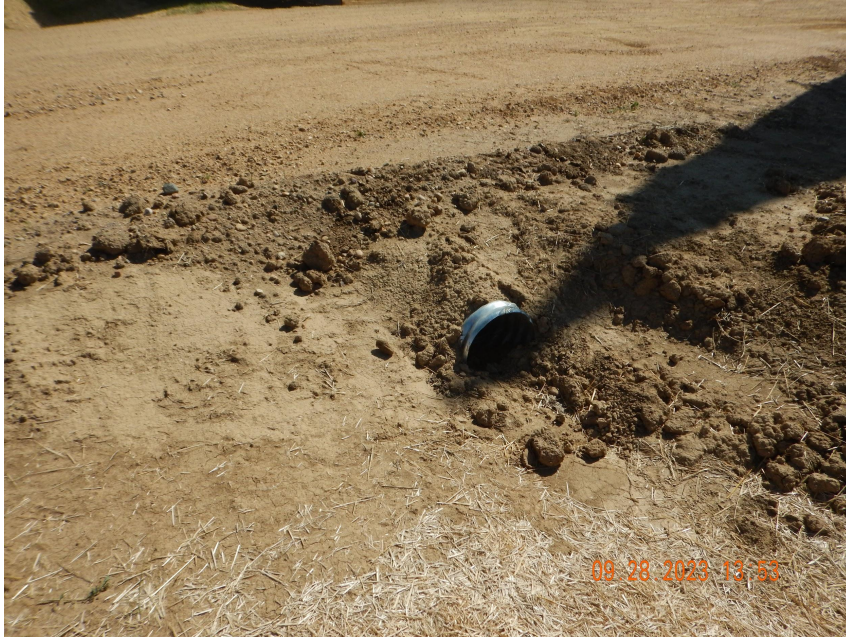
Photo 6. Photo taken from the northern perimeter of location and access road. Photo illustrates the culvert does not have any inlet or outlet protection.
