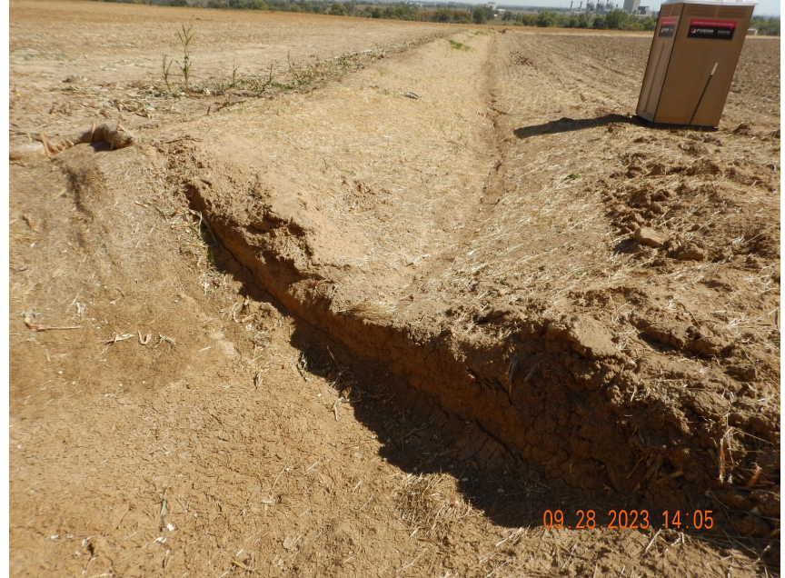
Photo 11. Photo taken from the eastern perimeter of location illustrating the 1:1 side slopes of the sediment trap which are not installed per good engineering practices.
