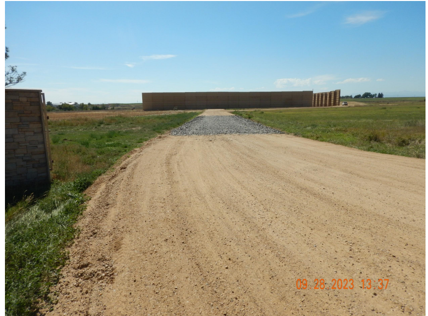
Photo 3. Photo taken from the entrance of location, facing South. Photo illustrates the Operator has installed a VTC device BMP which is in proper functioning at the of this inspection.
