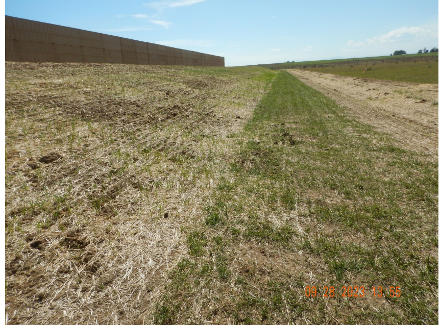
Photo 7. Photo taken from the northwestern perimeter of location, facing South. Photo illustrates the topsoil stockpile and stormwater BMPs areas have been seeded. Establishment of desirable vegetation was observed.
