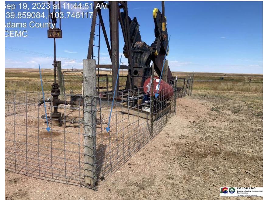
Pic 2 unused equipment / trash needs to be removed, stained soil needs to be removed.
