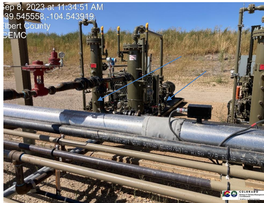
Pic 9 minor leak detected by CDPHE FLIR inspector.
