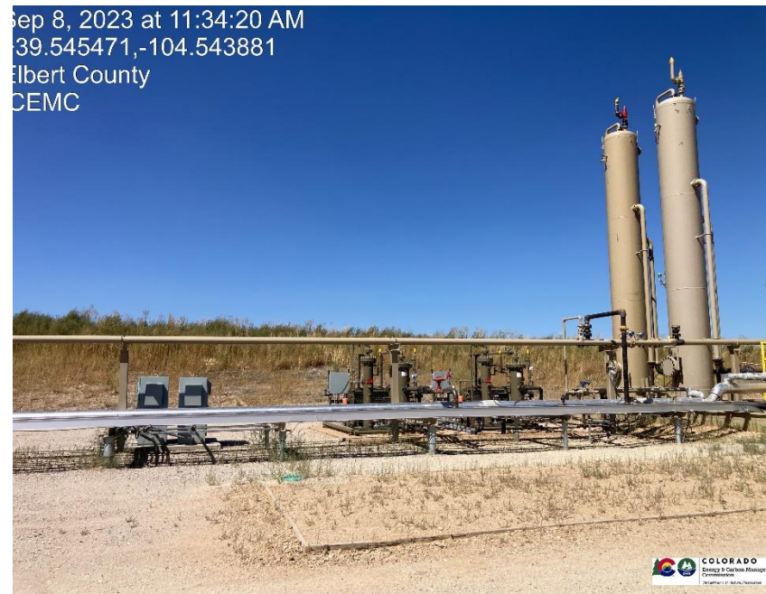
Pic 8 VRU, VRT, small leak detected by CDPHE FLIR inspection.
