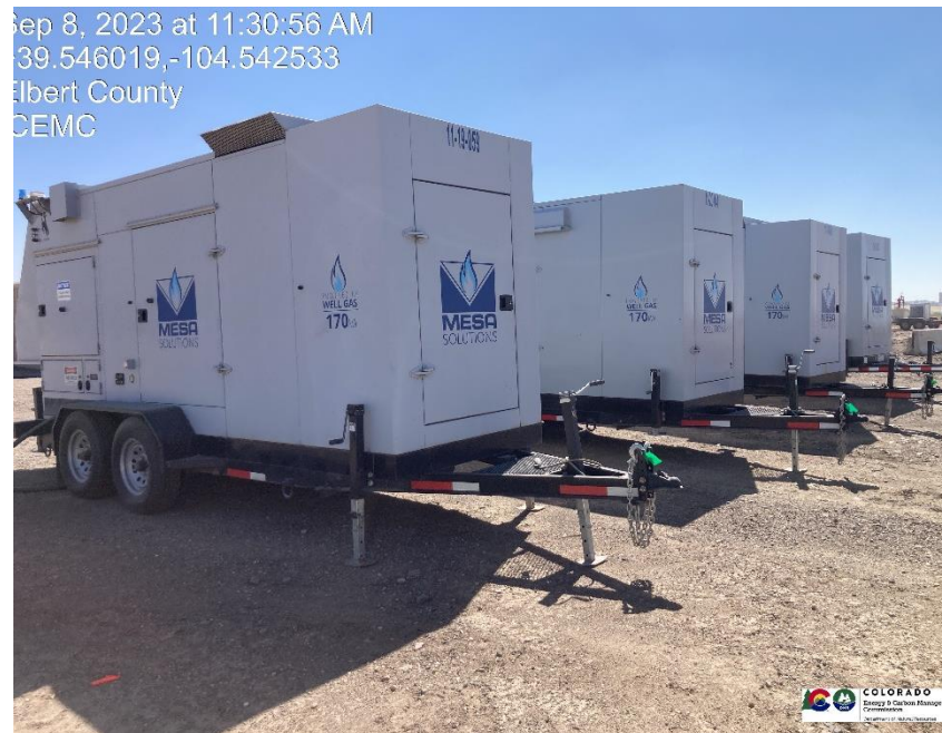
Pic 2 gas generators for ESP
