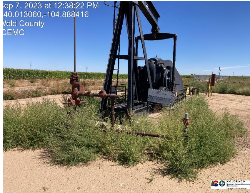
Pic 1 wellhead / pumpjack / weeds unmanged
