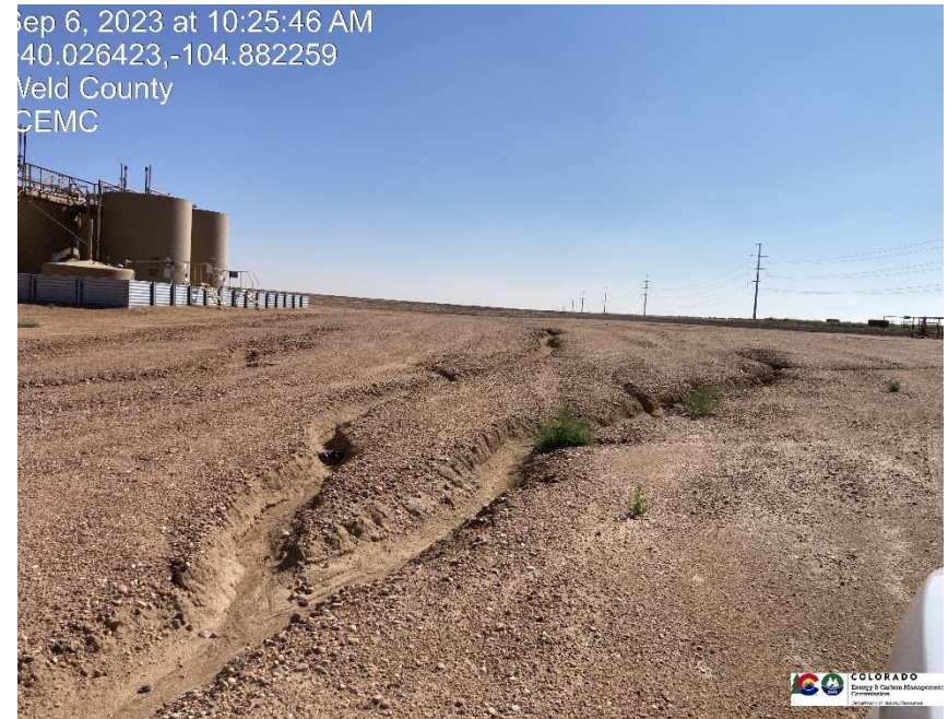
Pic 2 Erosion control measure failure
