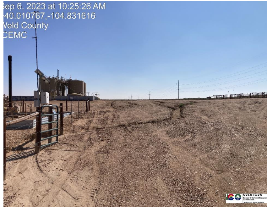
Pic 1 Erosion control measure failure
