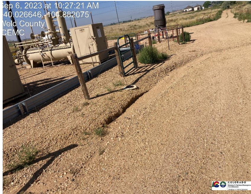
Pic 7 Stormwater control measure failure
