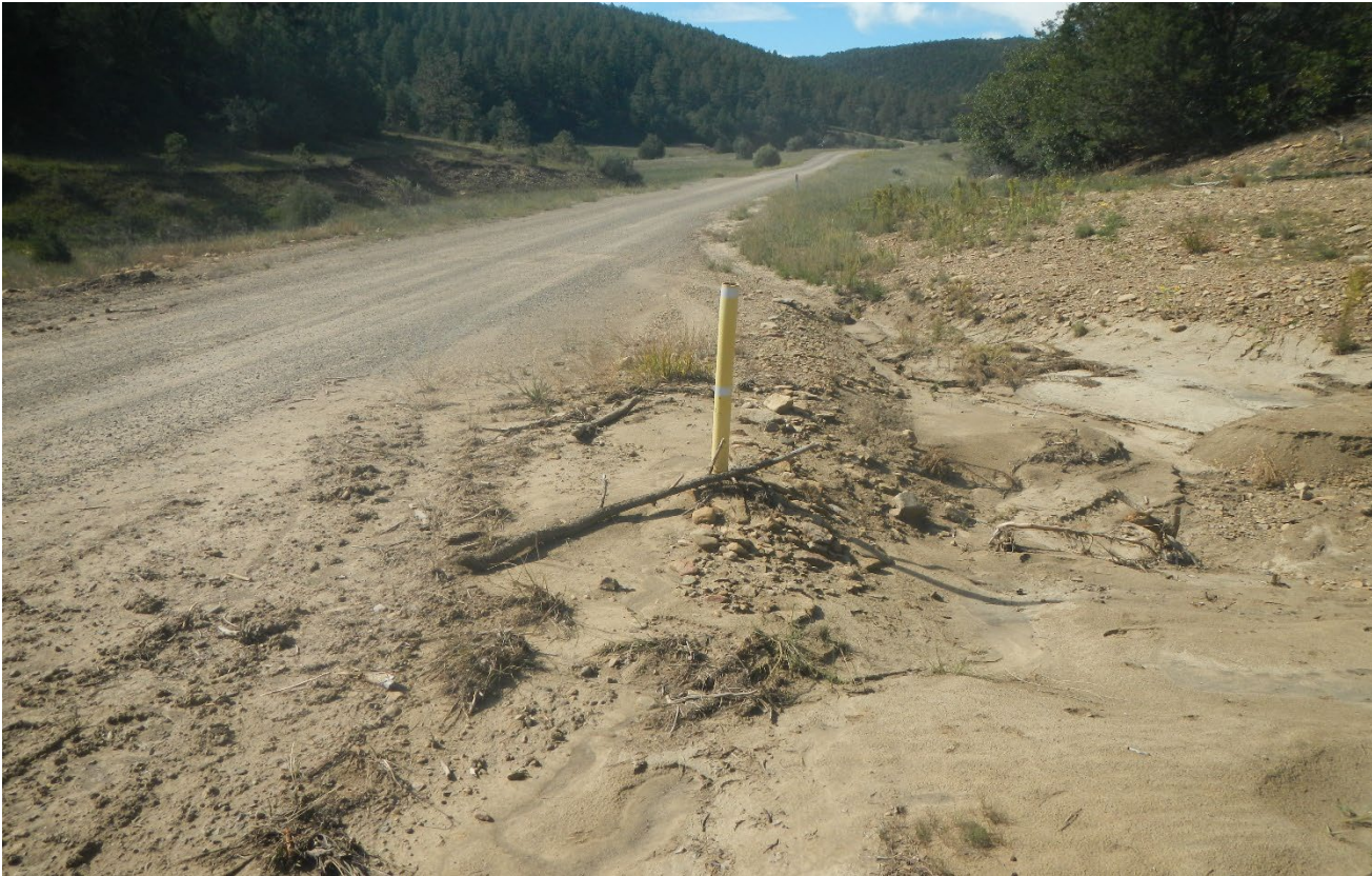
Photo 2. Facing west along the road. This culvert has filled in with sediment. Lat/Long:37.14485,-104.03594.
