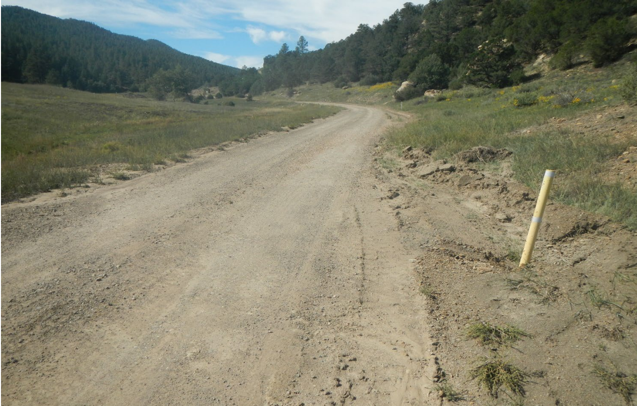
Photo 1. Facing west at the main access road. The road has been recently graded. This culvert is partially filled in with sediment.
