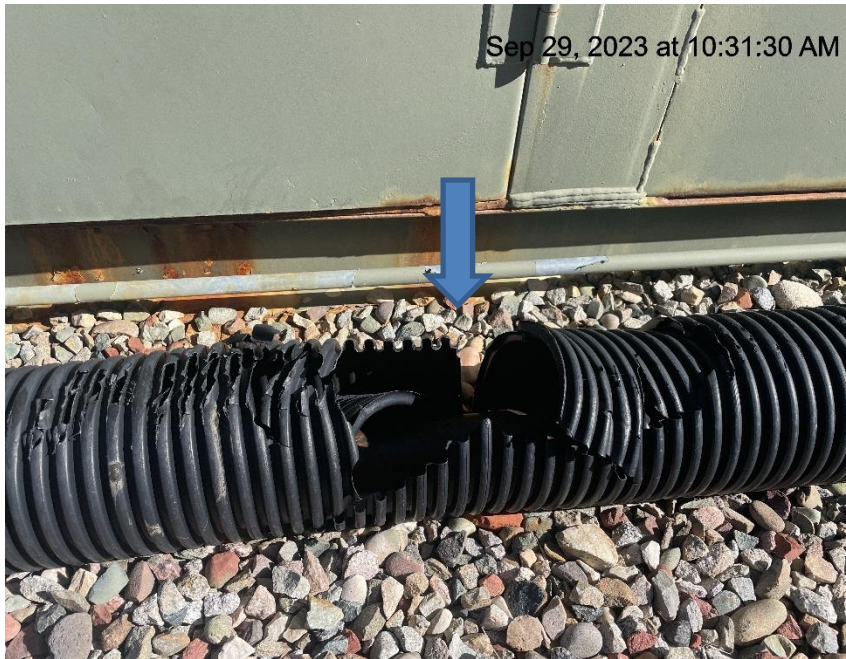
Photo # 977 Flowline heating insulation with a hole/wildlife hazard
