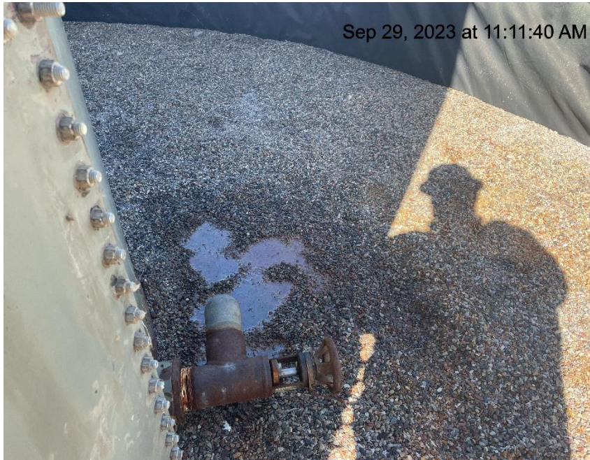
Photo # 1043 Leaking valve on production tank/stained gravel
