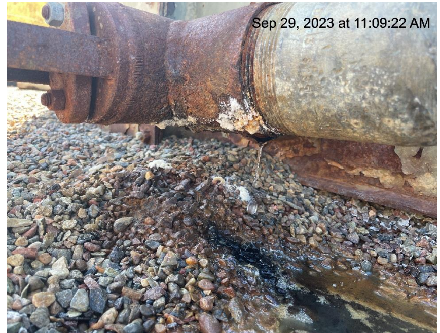
Photo # 1040 Fluid leaking from valve
