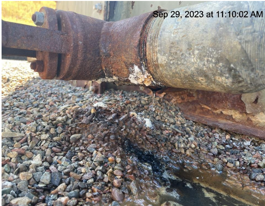
Photo # 1041 Fluid leaking from valve
