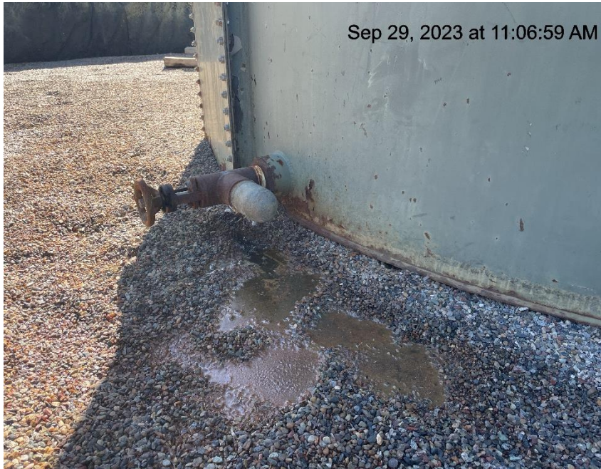
Photo # 1039 Leaking valve on production tank/stained gravel
