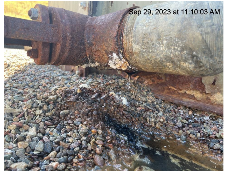
Photo # 1042 Fluid leaking from valve
