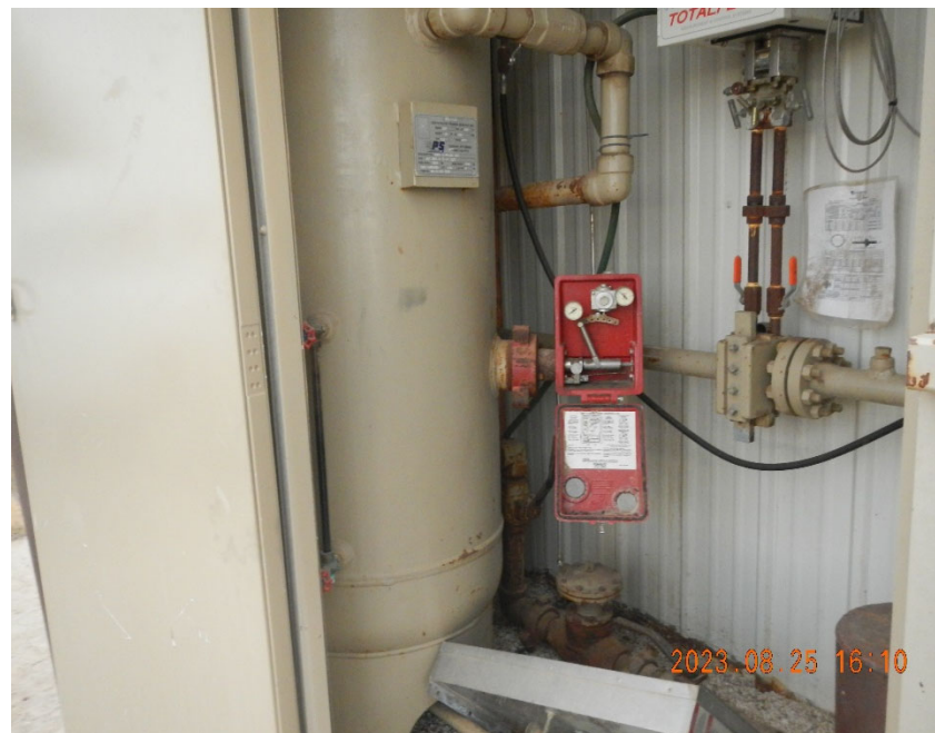
6. Vertical separator, digital meter and knock out vessel inside meter shed.
