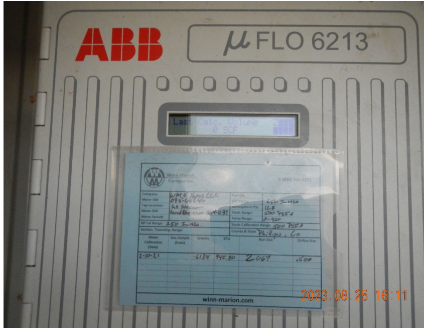
7. Meter Calibration/Test Log inside meter shed at time of inspection.
