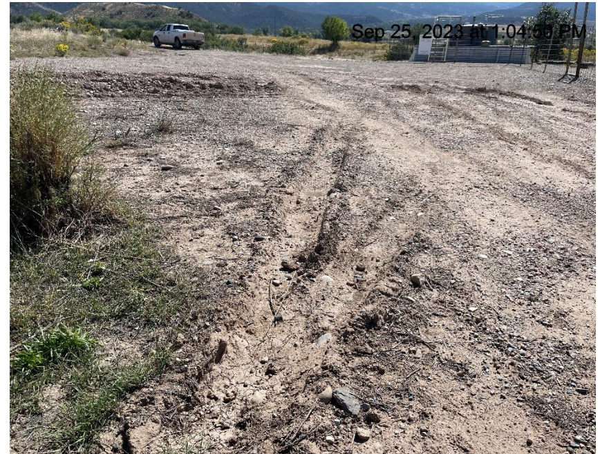
Photo # 793 Lack of stabilization/compaction on location /insufficient BMP's
