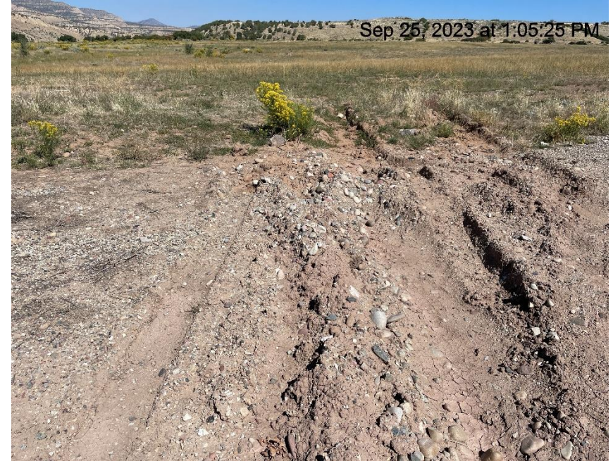
Photo # 795 Lack of stabilization/compaction on location /insufficient BMP's
