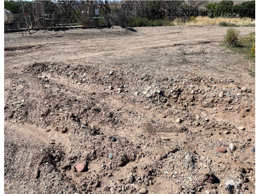
Photo # 799 Lack of stabilization/compaction on location /insufficient BMP's
