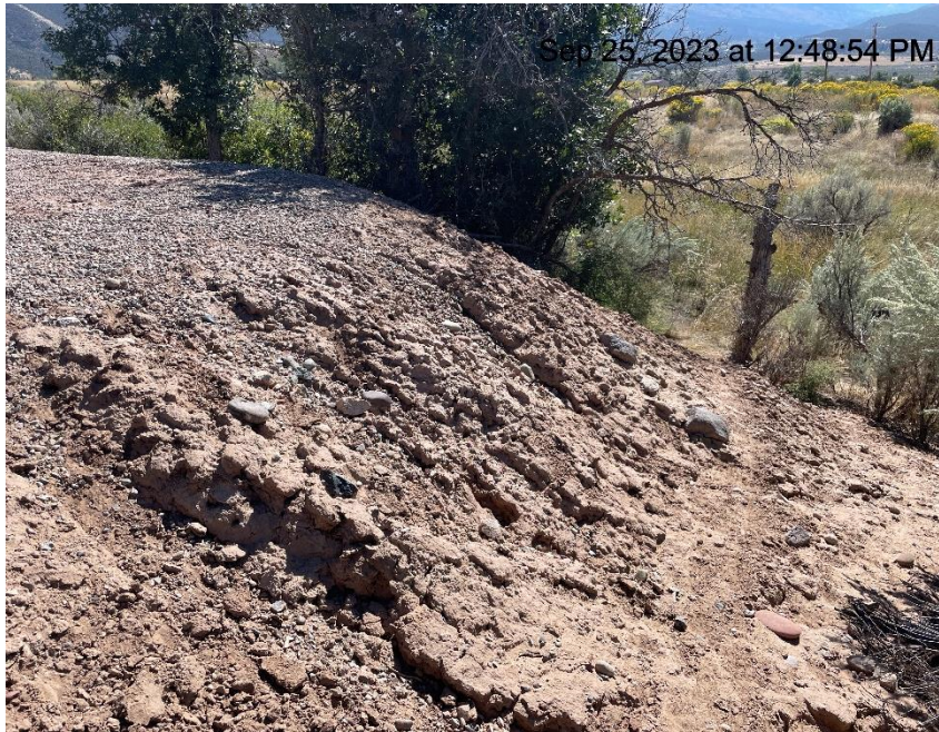
Photo # 774 Erosion on slope & transport of sediment off location/insufficient BMP's (S/SE area of location)
