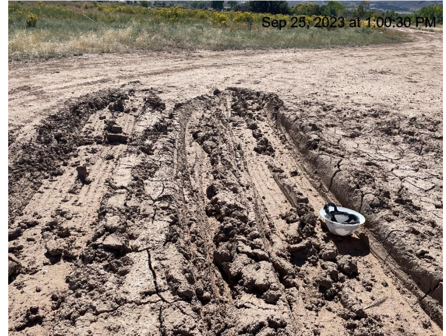
Photo # 785 Lack of stabilization/compaction on location /insufficient BMP's
