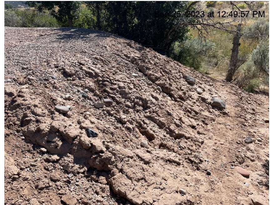
Photo # 775 Erosion on slope & transport of sediment off location/insufficient BMP's (S/SE area of location)
