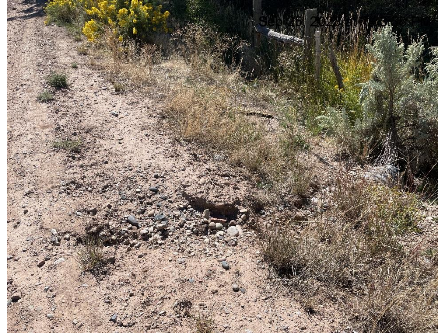
Photo # 781 Erosion & transport of sediment off lease road (on short portion of lease road between production equipment & wellheads, near culvert)
