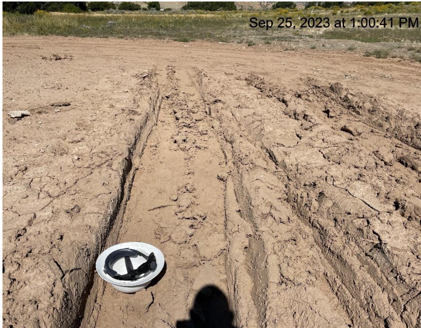
Photo # 786 Lack of stabilization/compaction on location /insufficient BMP's
