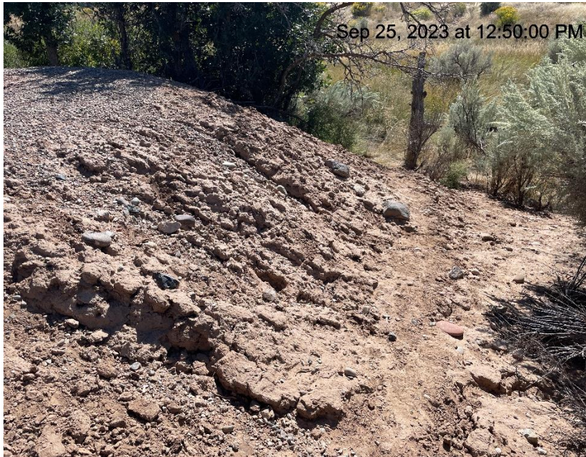
Photo # 776 Erosion on slope & transport of sediment off location/insufficient BMP's (S/SE area of location)
