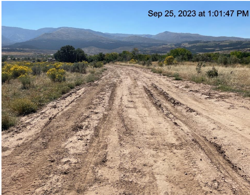
Photo # 790 Lack of stabilization/compaction on lease road /insufficient BMP's
