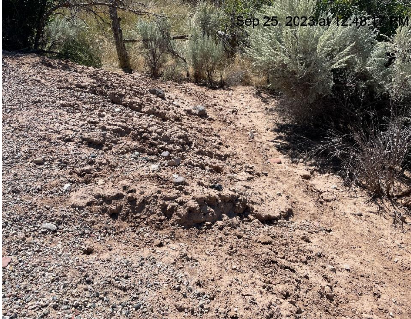
Photo # 770 Erosion on slope & transport of sediment off location/insufficient BMP's (S/SE area of location)
