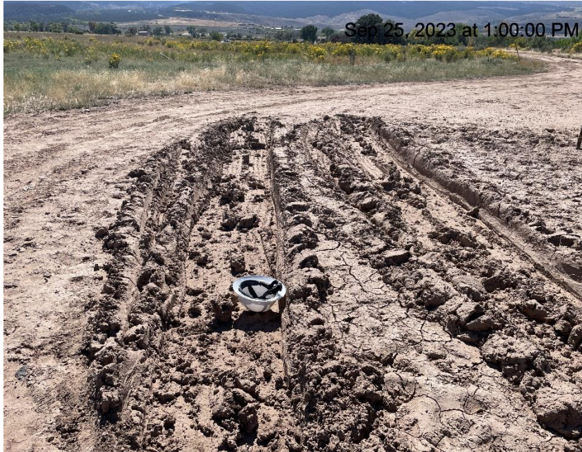
Photo # 784 Lack of stabilization/compaction on location /insufficient BMP's
