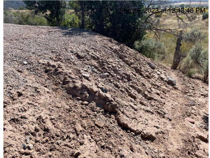
Photo # 773 Erosion on slope & transport of sediment off location/insufficient BMP's (S/SE area of location)
