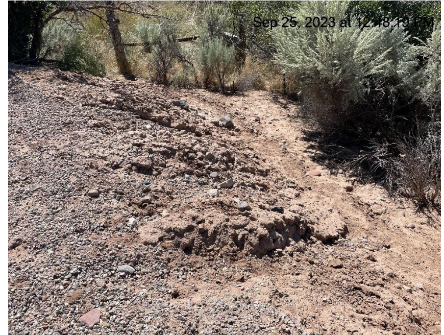
Photo # 771 Erosion on slope & transport of sediment off location/insufficient BMP's (S/SE area of location)
