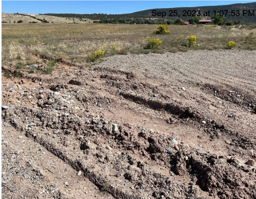
Photo # 800 Lack of stabilization/compaction on location /insufficient BMP's
