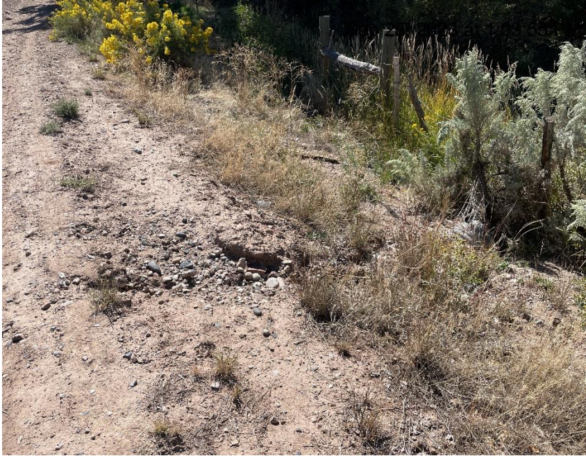
Photo # 780 Erosion & transport of sediment off lease road (on short portion of lease road between production equipment & wellheads, near culvert)
