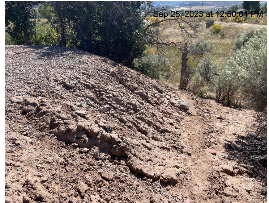
Photo # 777 Erosion on slope & transport of sediment off location/insufficient BMP's (S/SE area of location)
