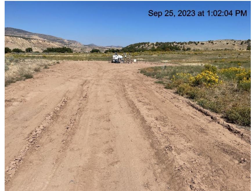
Photo # 791 Lack of stabilization/compaction on lease road /insufficient BMP's
