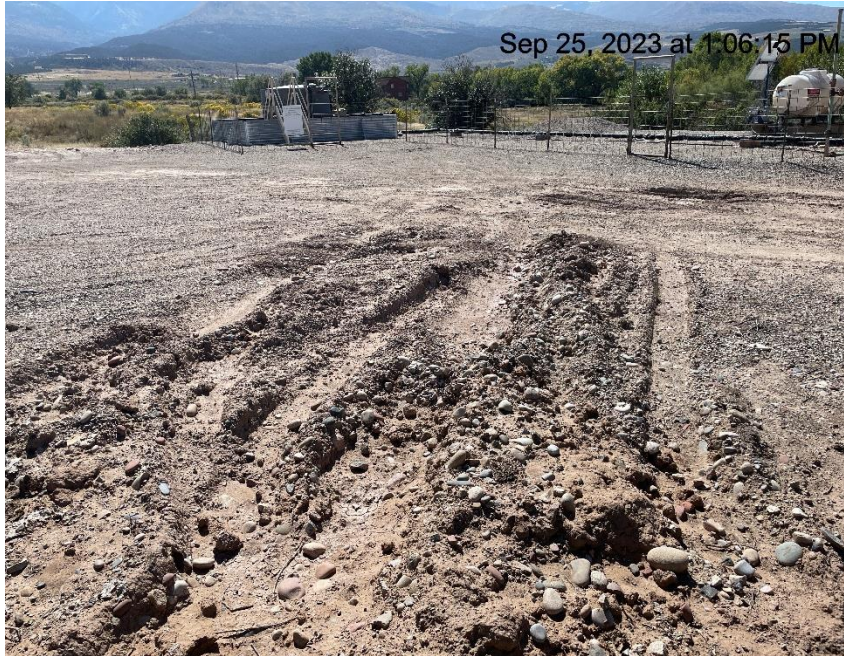
Photo # 798 Lack of stabilization/compaction on location /insufficient BMP's
