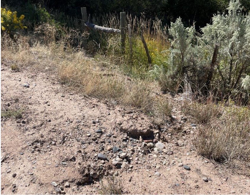
Photo # 778 Erosion & transport of sediment off lease road (on short portion of lease road between production equipment & wellheads, near culvert)
