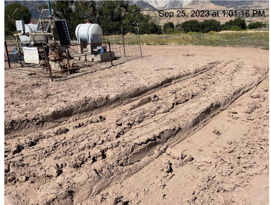
Photo # 789 Lack of stabilization/compaction on location /insufficient BMP's
