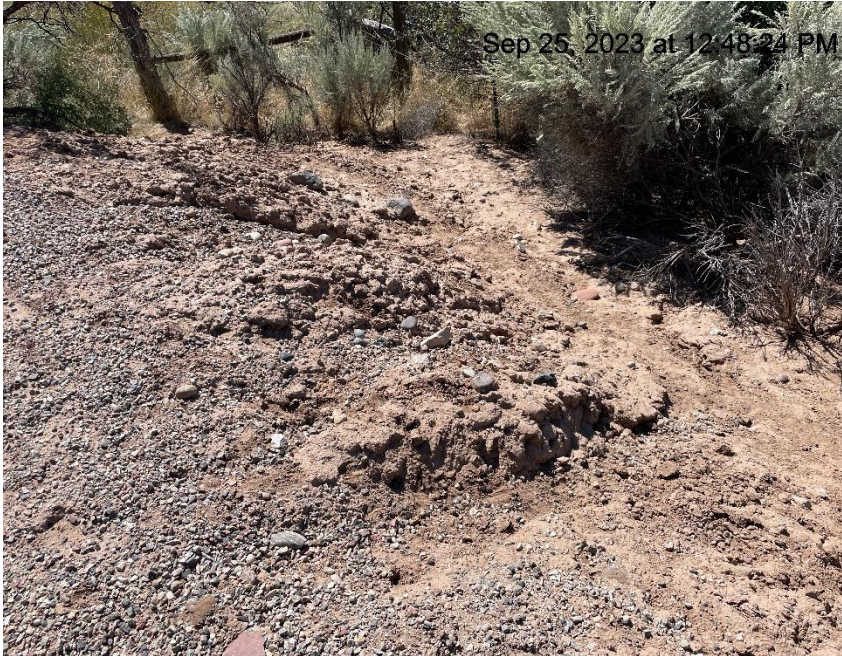
Photo # 772 Erosion on slope & transport of sediment off location/insufficient BMP's (S/SE area of location)
