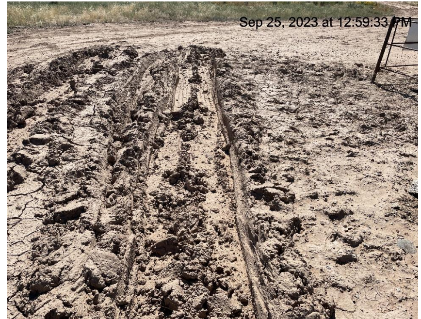
Photo # 783 Lack of stabilization/compaction on location /insufficient BMP's
