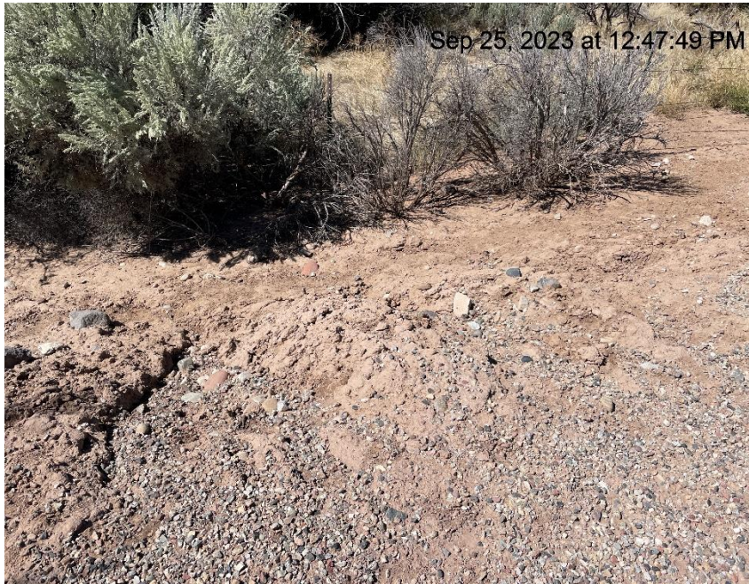
Photo # 768 Erosion on slope & transport of sediment off location/insufficient BMP's (S/SE area of location)
