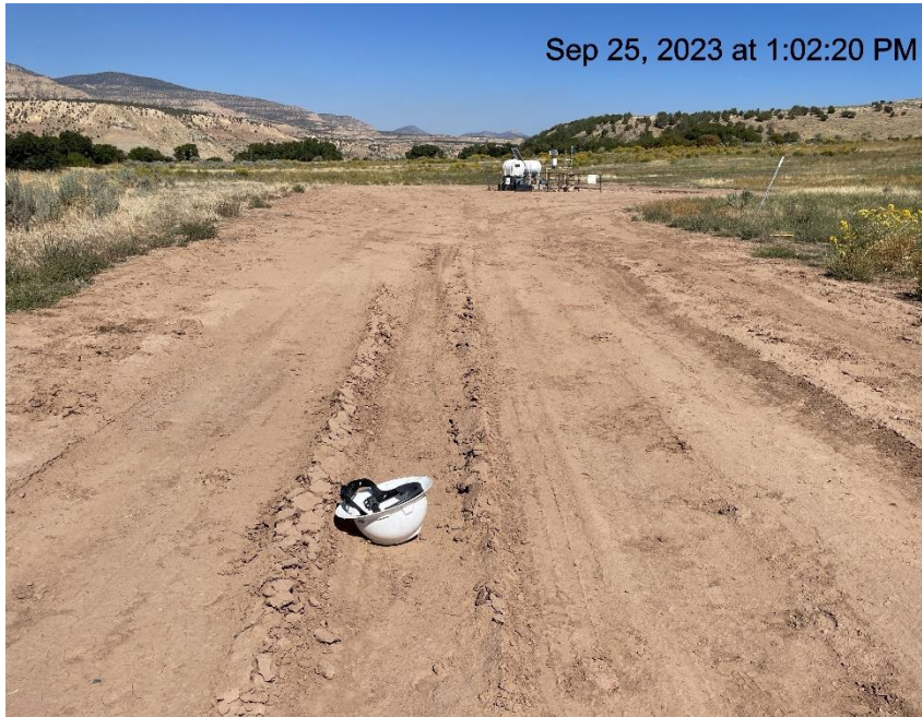
Photo # 792 Lack of stabilization/compaction on lease road /insufficient BMP's
