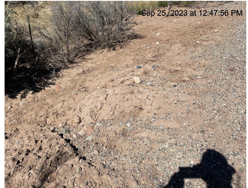
Photo # 769 Erosion on slope & transport of sediment off location/insufficient BMP's (S/SE area of location)
