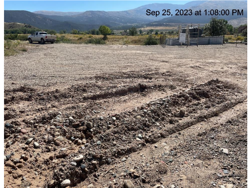
Photo # 801 Lack of stabilization/compaction on location /insufficient BMP's
