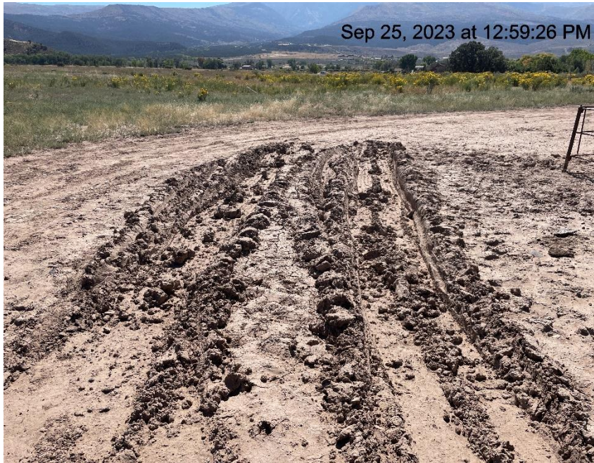
Photo # 782 Lack of stabilization/compaction on location /insufficient BMP's
