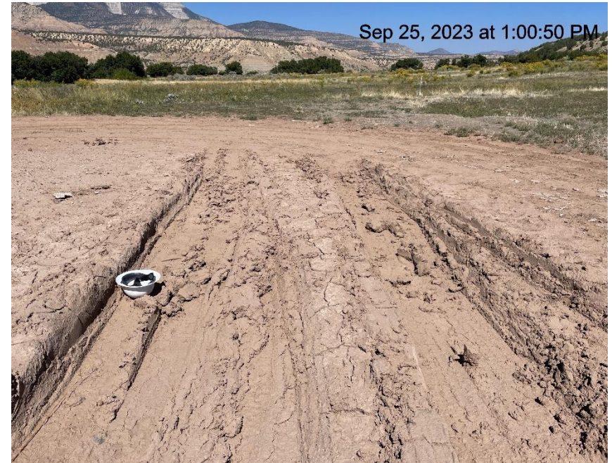
Photo # 787 Lack of stabilization/compaction on location /insufficient BMP's
