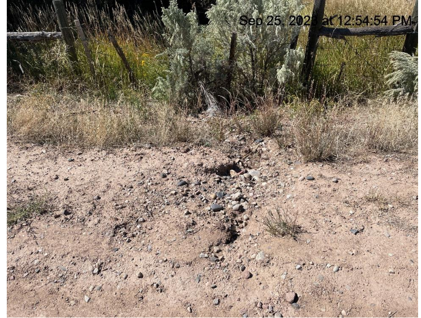
Photo # 779 Erosion & transport of sediment off lease road (on short portion of lease road between production equipment & wellheads, near culvert)
