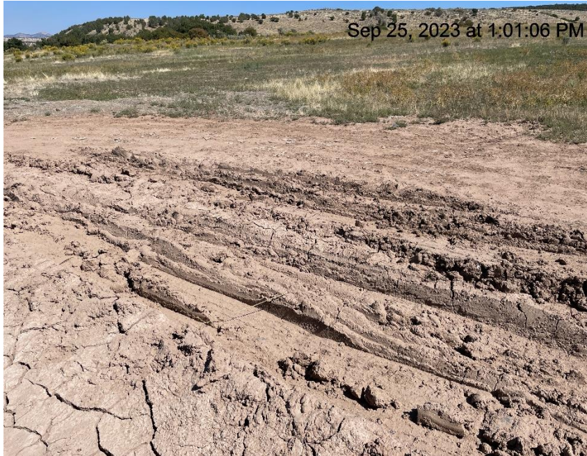
Photo # 788 Lack of stabilization/compaction on location /insufficient BMP's
