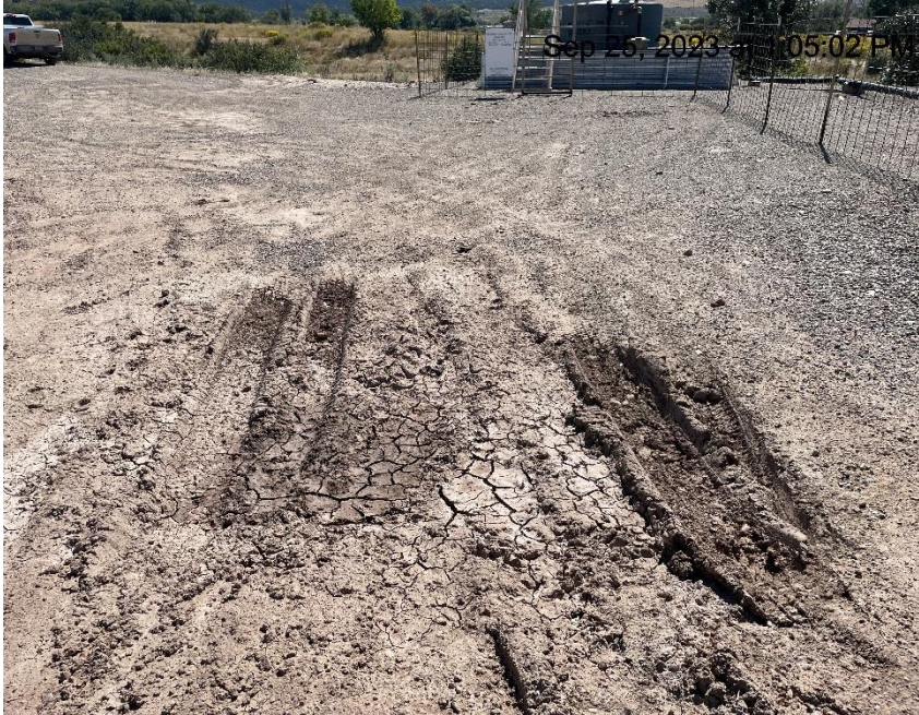
Photo # 794 Lack of stabilization/compaction on location /insufficient BMP's
