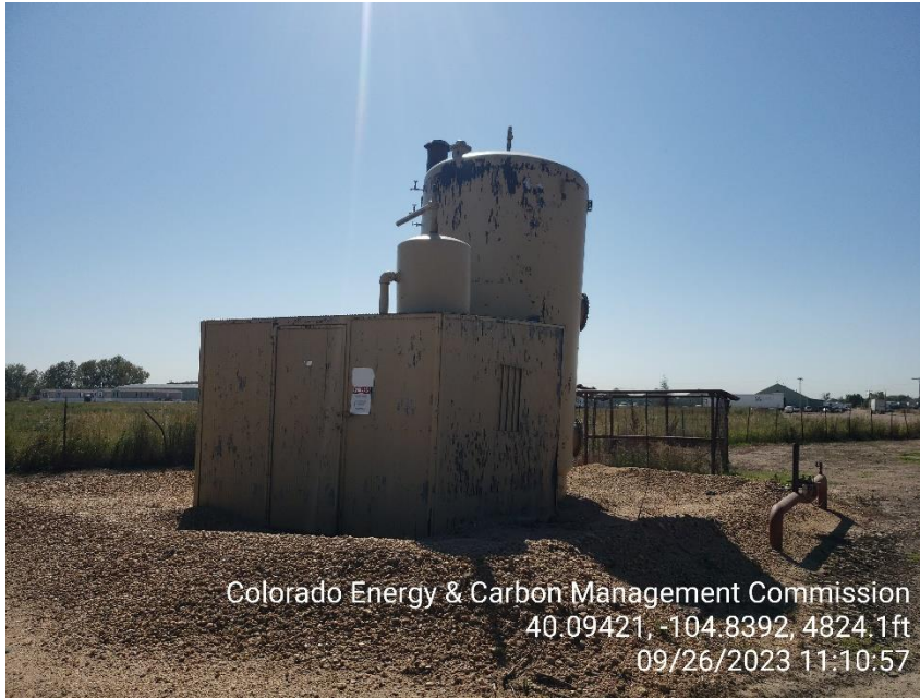
Photo 5 Vertical Heater Treater
