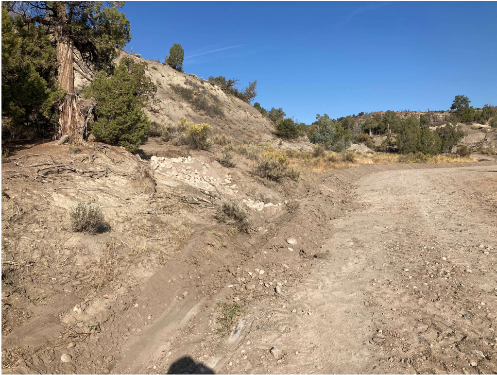
Repaired and reinforced overwhelmed ditch and Berm along west side of location
