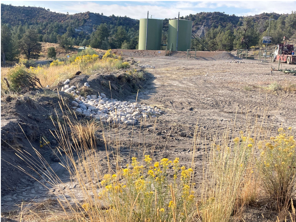
Installed and repaired BPMs on eastern side of location and mitigated sediment migration off location
