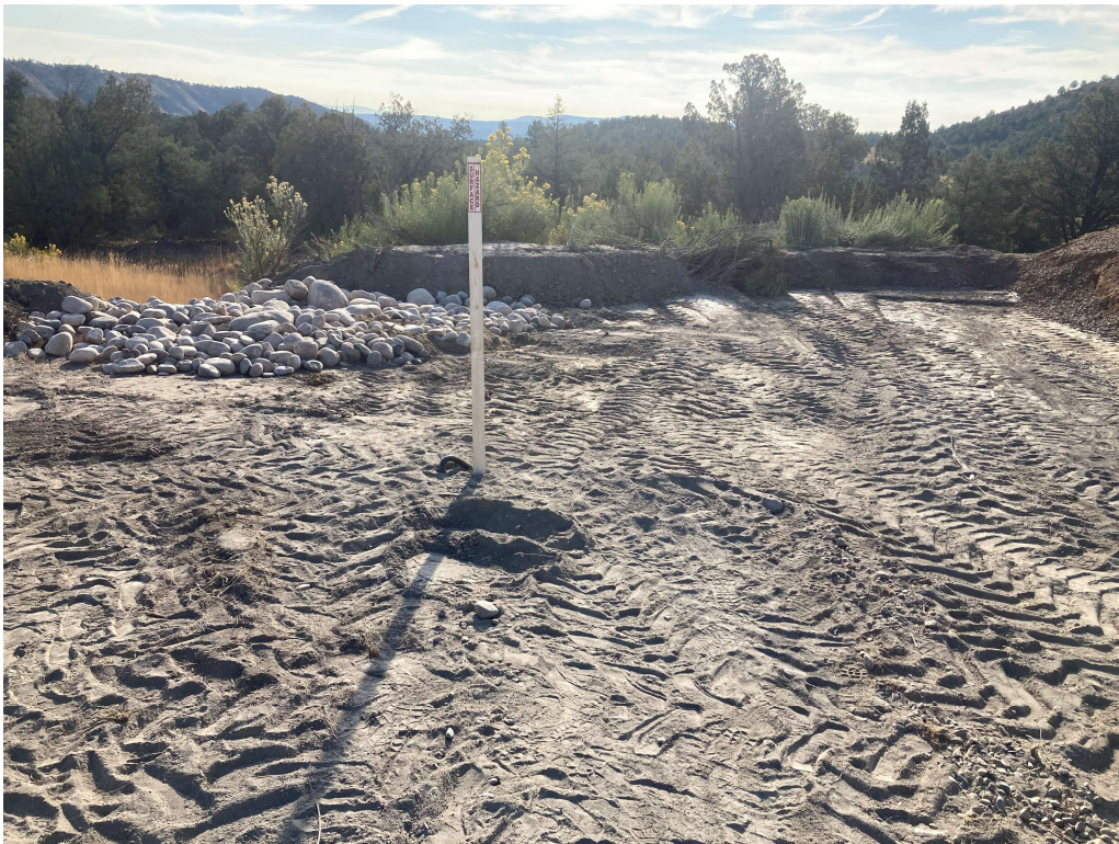
Marked all rig anchors on location
