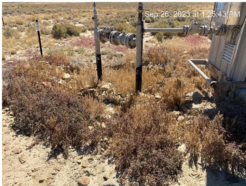
Erosion and sediment migration leaving location as in previous inspection
