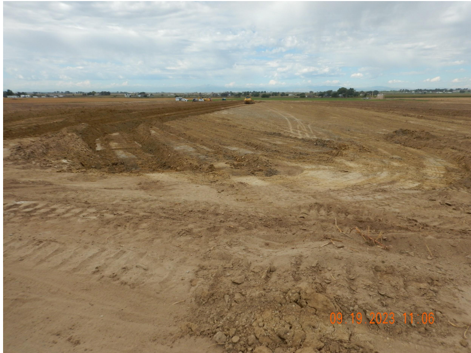
Photo 7. Photo taken from the eastern perimeter of location, facing West. Photo illustrates Operator is completing the cut/fill construction phase. Topsoil has been stockpiled along the southern, eastern and northern perimeter of the location.
