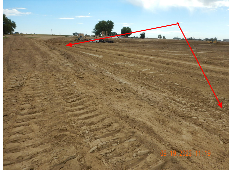
Photo 10. Photo taken from the northern perimeter of location, facing East. Photo illustrates a diversion ditch BMP installed along the perimeter of the working pad surface which is directed to detention pond.
