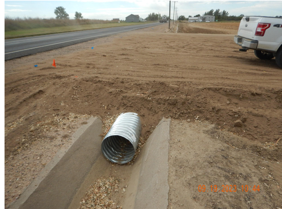
Photo 2. Photo taken from the location entrance, facing South. Photo illustrates culvert has been installed and BMP installation is in-process. Operator plans to install inlet and outlet protection devices. Operator also plans to install recycled asphalt at the location entrance and to install additional VTC devices.
