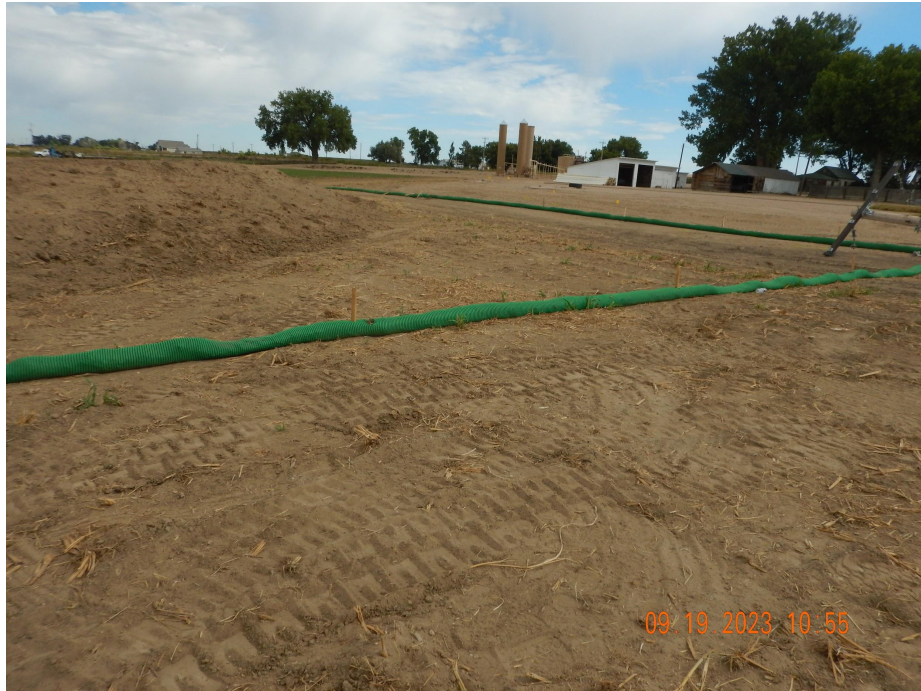
Photo 5. Photo taken from the southeastern perimeter of location, facing Northeast. Photo illustrates Operator has installed filterx wattles as an initial BMP around the perimeter of the location.
