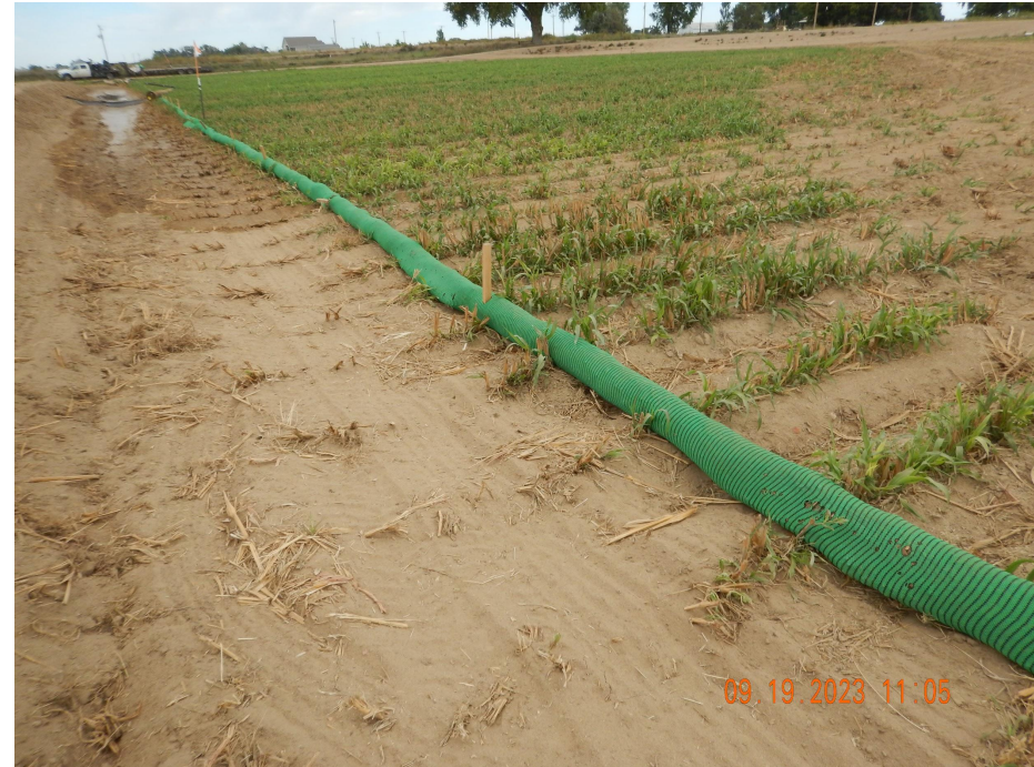
Photo 6. Photo taken from the eastern perimeter of location, facing Northeast. Photo illustrates Operator has improperly installed filterx wattles as an initial BMP intended for run-on protection.
