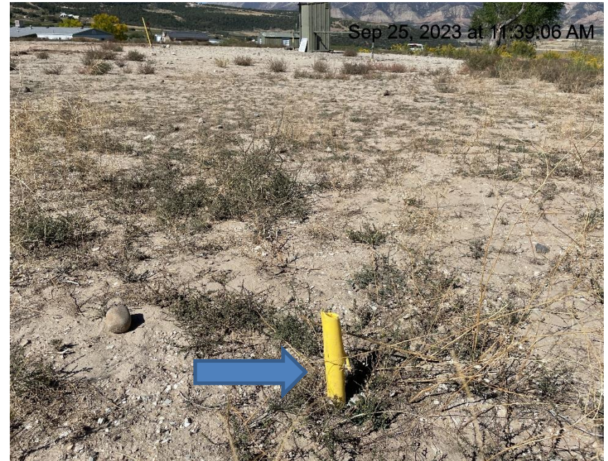
Photo # 642 Improperly marked deadman
