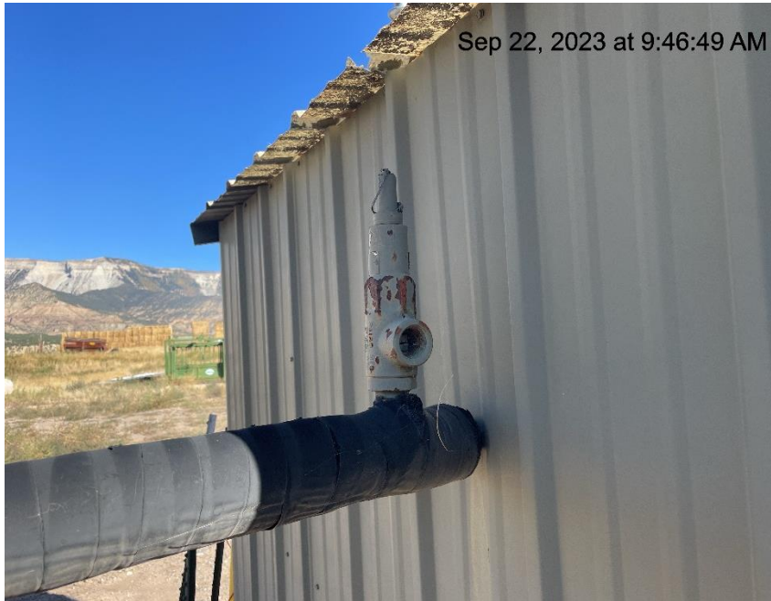
Photo # 126 PRV lacks vent line
