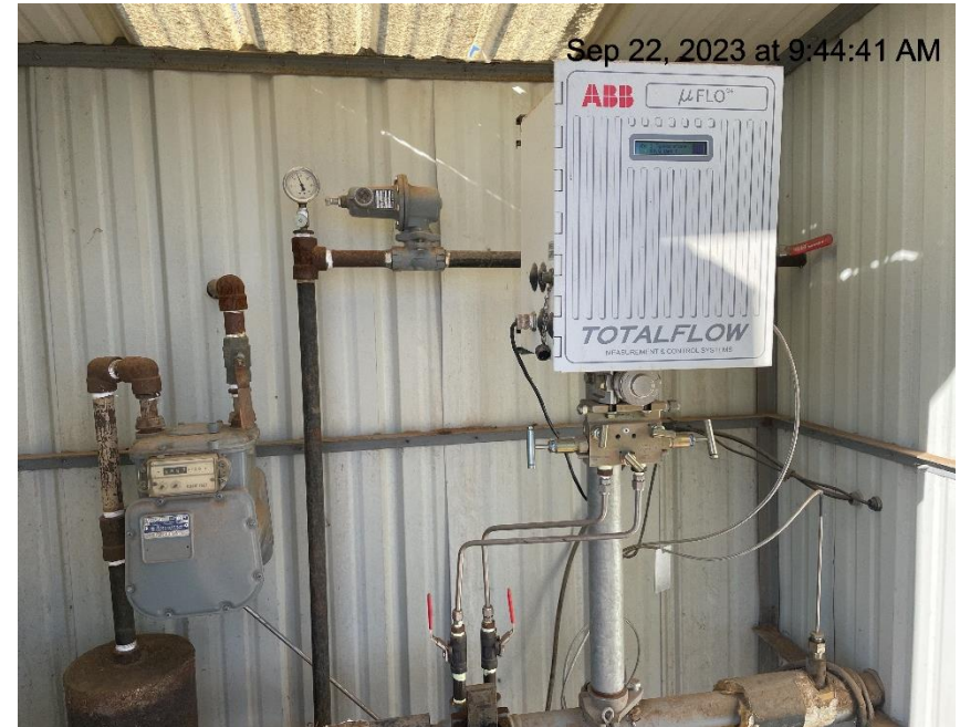
Photo # 123 Meter calibration info not conspicuously posted
