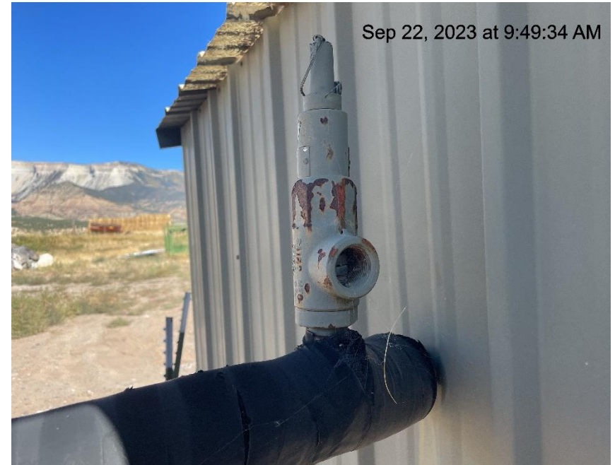
Photo # 127 PRV lacks vent line
