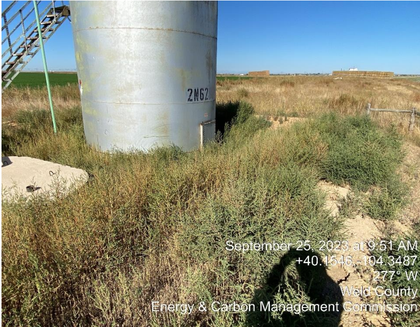
Missing Capacity Label & Overgrown Vegetation
