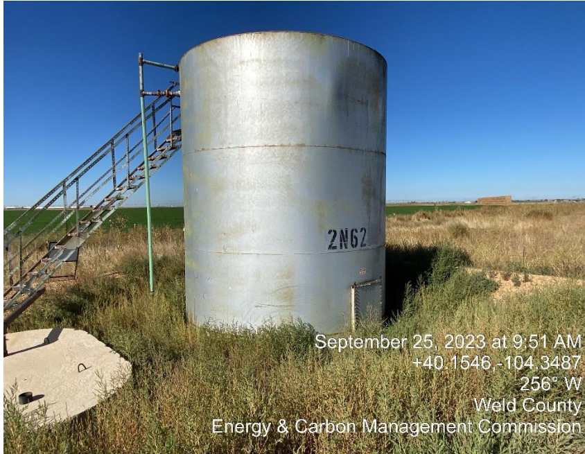
Missing Capacity Label & Overgrown Vegetation
