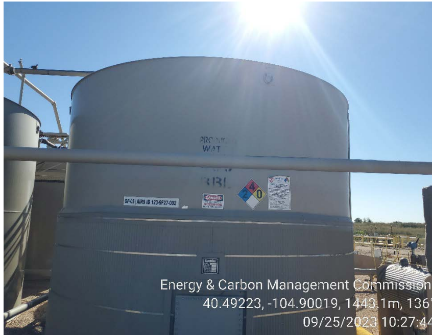
Produced water tank placards
