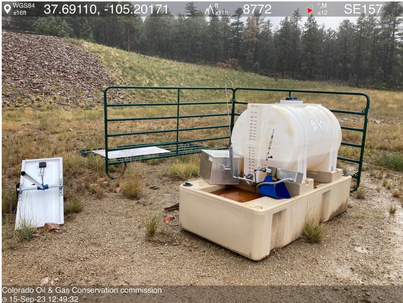
PHOTO 4: There is no labeling at the chemical tank next to the well. Install sign to comply with Rule 605.h. THIS IS THE SECOND NOTICE OF THIS CORRECTIVE ACTION, IMMEDIATE ACTION IS REQUIRED.
