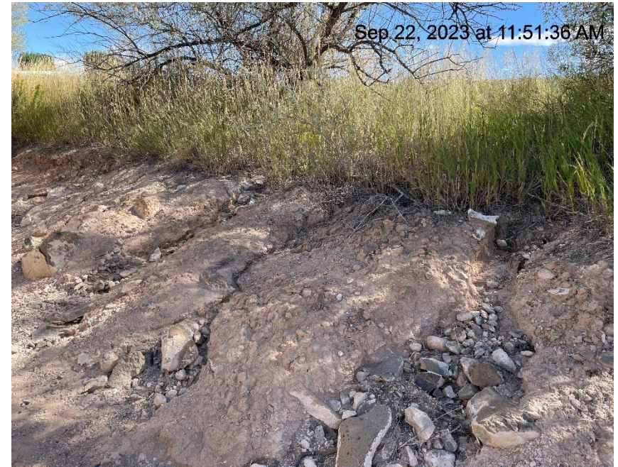
Photo # 388 Erosion & transport of sediment onto location/ insufficient BMP's
