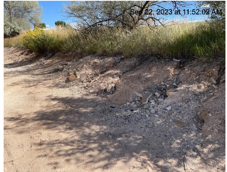
Photo # 394 Erosion & transport of sediment onto location/ insufficient BMP's
