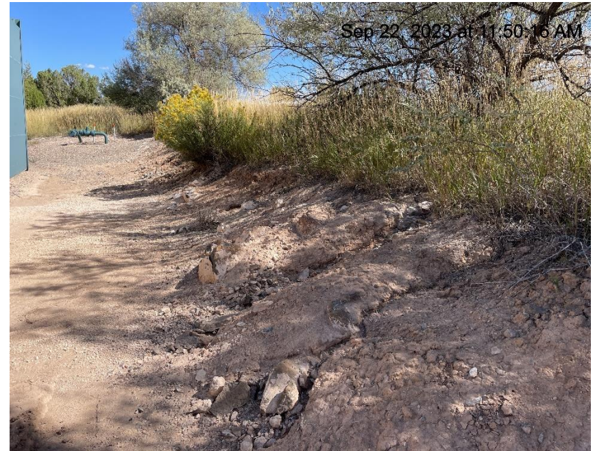
Photo # 365 Erosion & transport of sediment onto location/ insufficient BMP's
