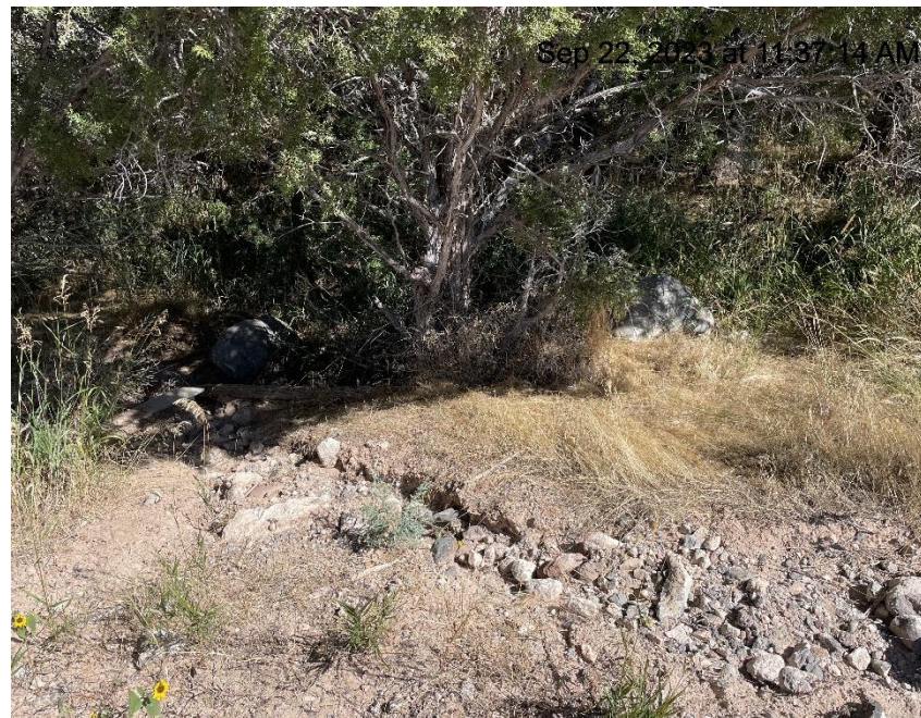
Photo # 346 Erosion & transport of sediment off location & into a vegetated area
