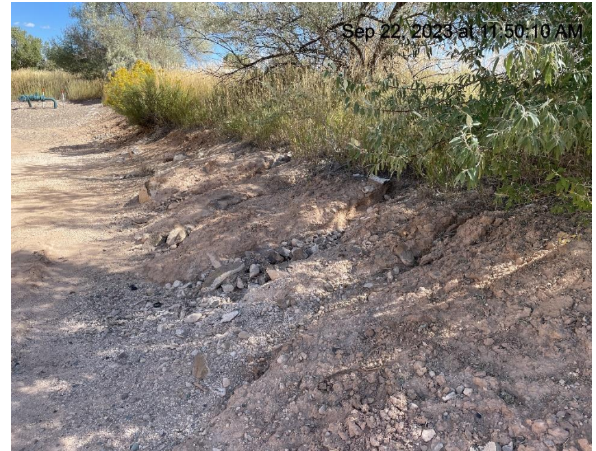
Photo # 363 Erosion & transport of sediment onto location/ insufficient BMP's
