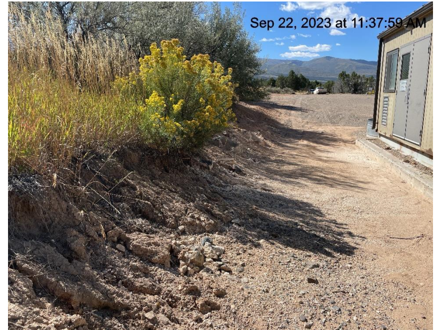
Photo # 349 Lack of stabilization & erosion on slope /transport of sediment onto location/insufficient BMP's
