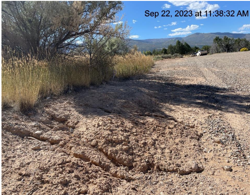
Photo # 356 Erosion & transport of sediment onto location/ insufficient BMP's
