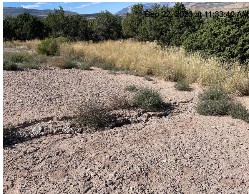
Photo # 317 Erosion & transport of sediment off location & into a vegetated area (W/NW area of location)
