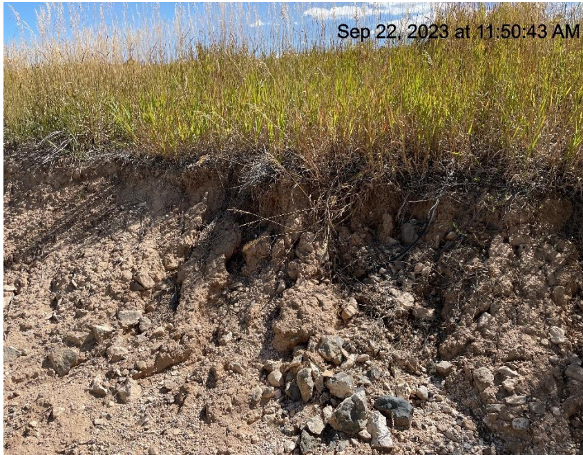
Photo # 373 Lack of stabilization & erosion on slope /transport of sediment onto location/insufficient BMP's
