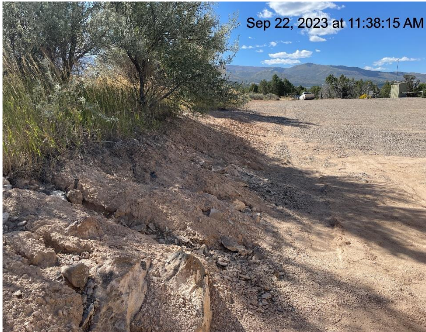
Photo # 352 Erosion & transport of sediment onto location/ insufficient BMP's
