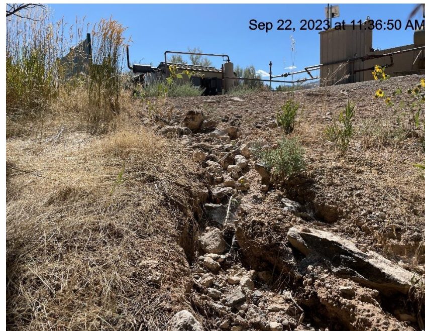
Photo # 342 Erosion & transport of sediment off location & into a vegetated area
