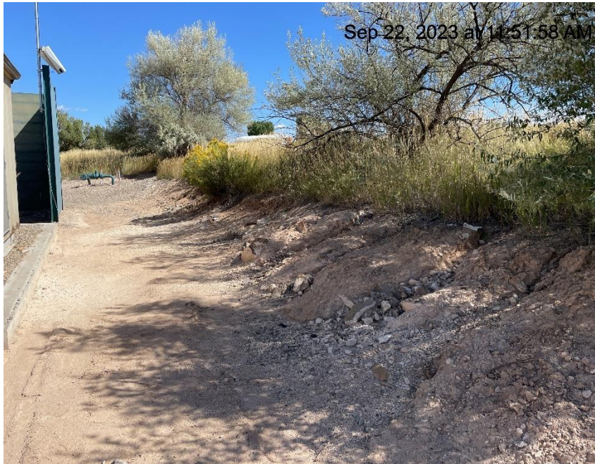
Photo # 393 Erosion & transport of sediment onto location/ insufficient BMP's
