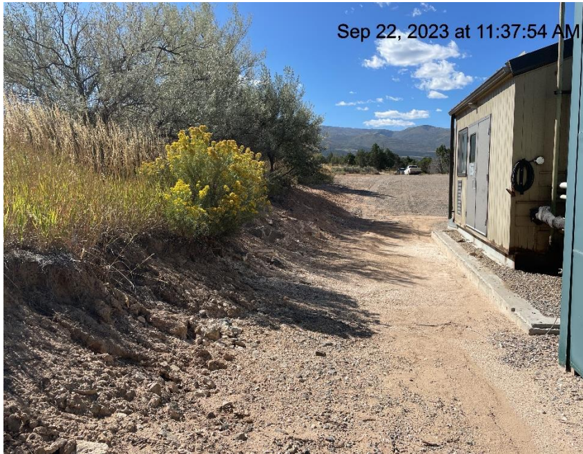
Photo # 348 Lack of stabilization & erosion on slope /transport of sediment onto location/insufficient BMP's
