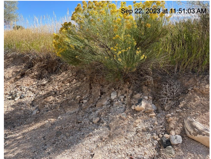
Photo # 378 Lack of stabilization & erosion on slope /transport of sediment onto location/insufficient BMP's
