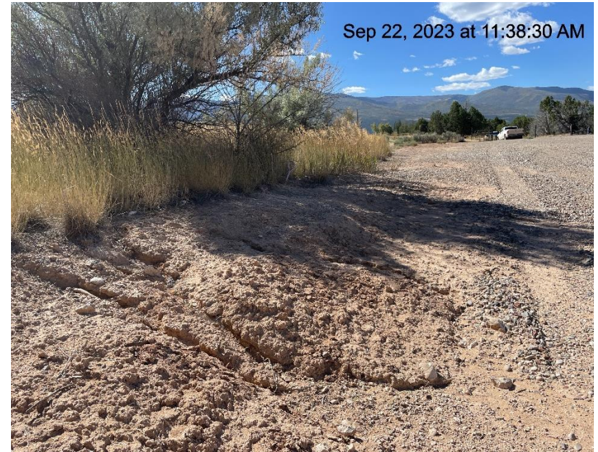
Photo # 355 Erosion & transport of sediment onto location/ insufficient BMP's
