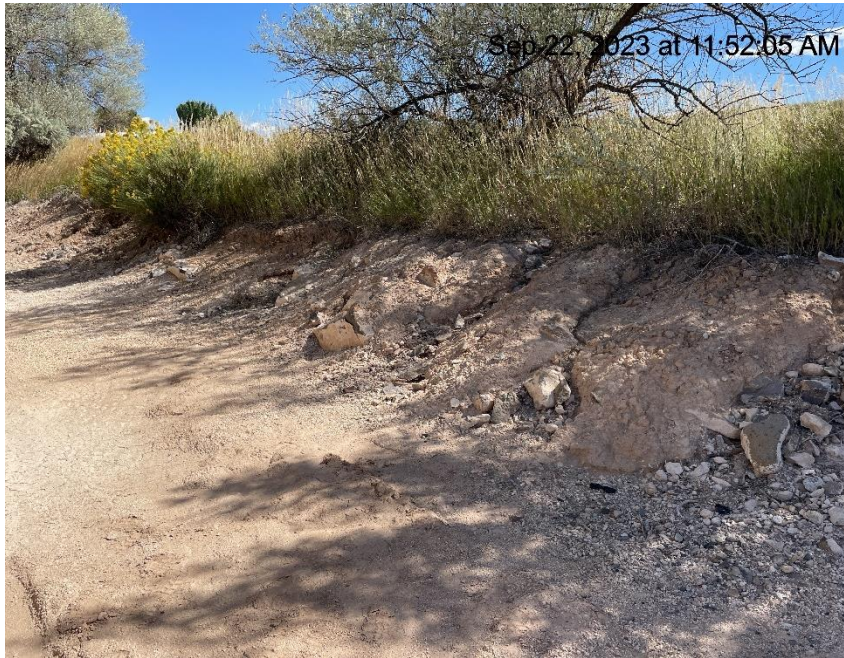
Photo # 395 Erosion & transport of sediment onto location/ insufficient BMP's
