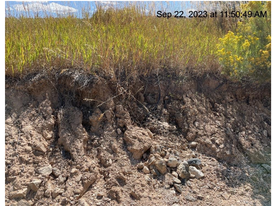
Photo # 375 Lack of stabilization & erosion on slope /transport of sediment onto location/insufficient BMP's
