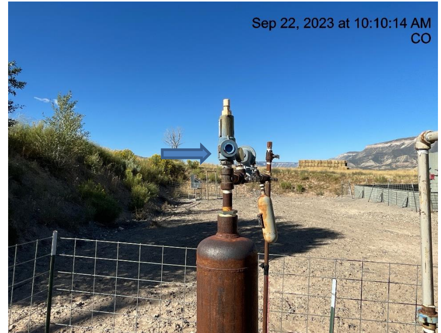
Photo # 163 PRV has plastic in relief port & no vent line
