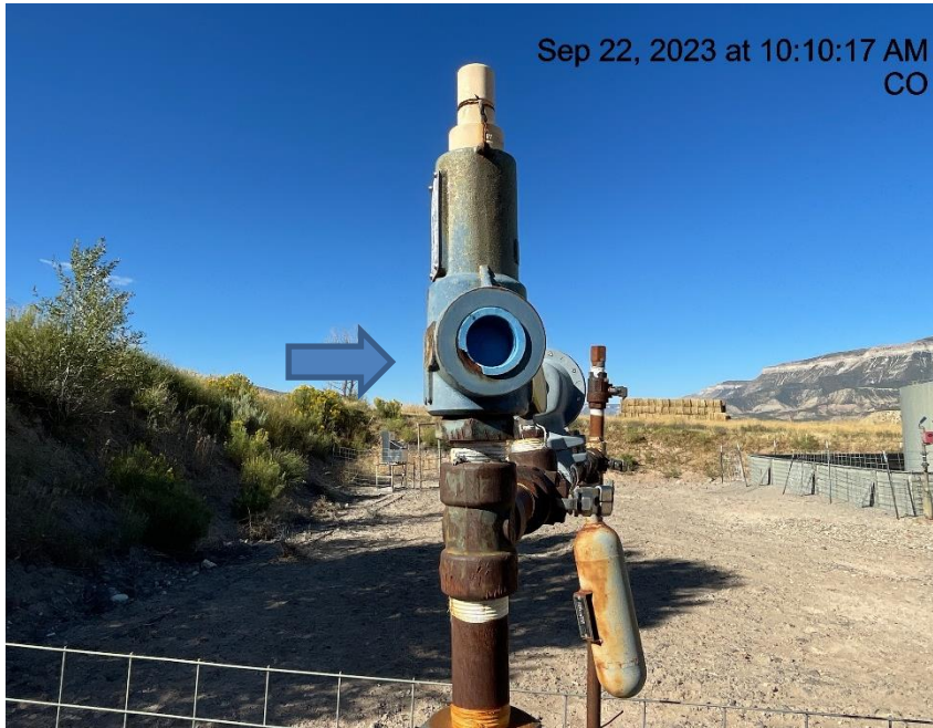
Photo # 164 PRV has plastic in relief port & no vent line
